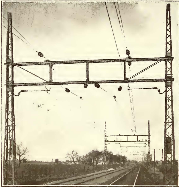
Dessau-Bitterfeld Railway—Construction at the End of a Tension-Regulating Section
