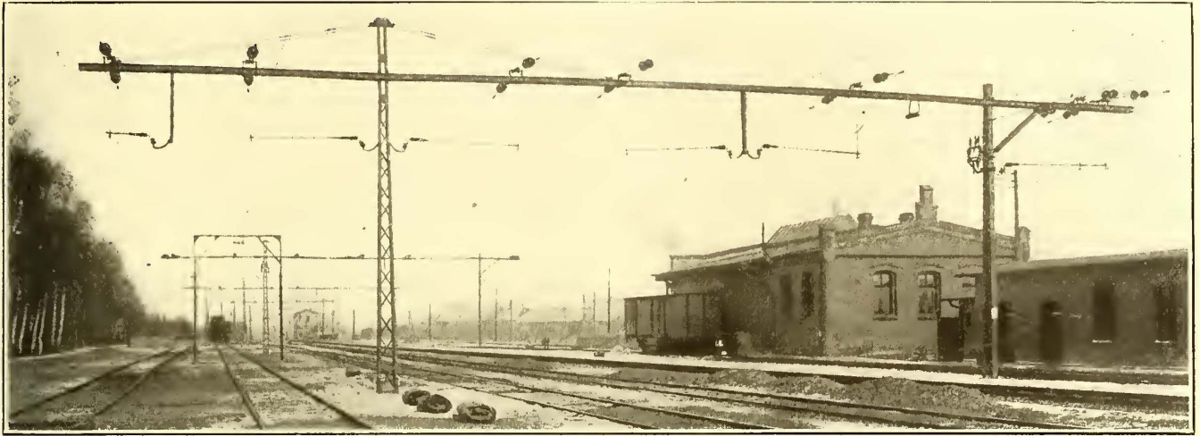
Dessau-Bitterfeld Railway—Overhead Construction for Six Tracks at Jessnitz
