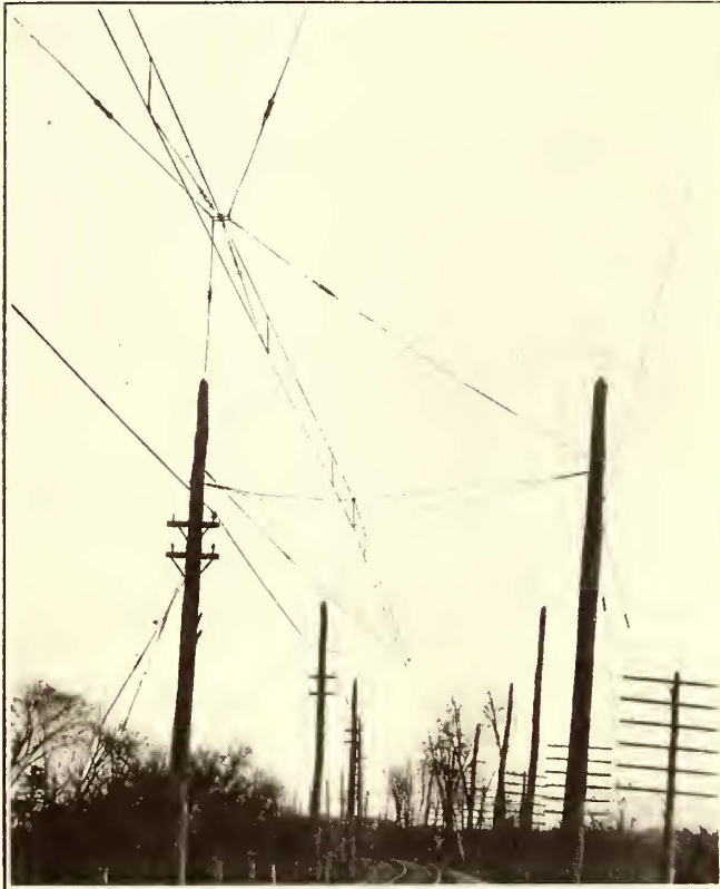
Catenary Lines After Test—View of Anchorage on Section of Span Construction
