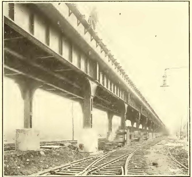
Hudson Tunnel Traffic—Elevated Structure in Newark
