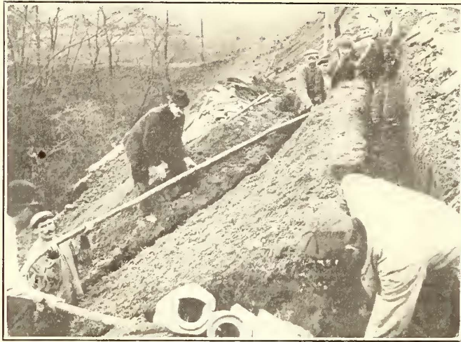
A Turn in the High-Tension Cable
