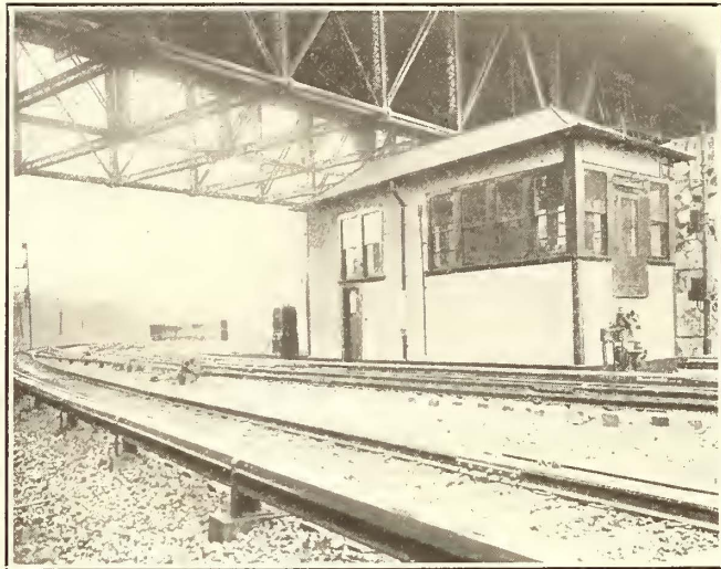
Hudson Tunnel Traffic—Interlocking Tower at Tunnel Portal on Pennsylvania Railroad
