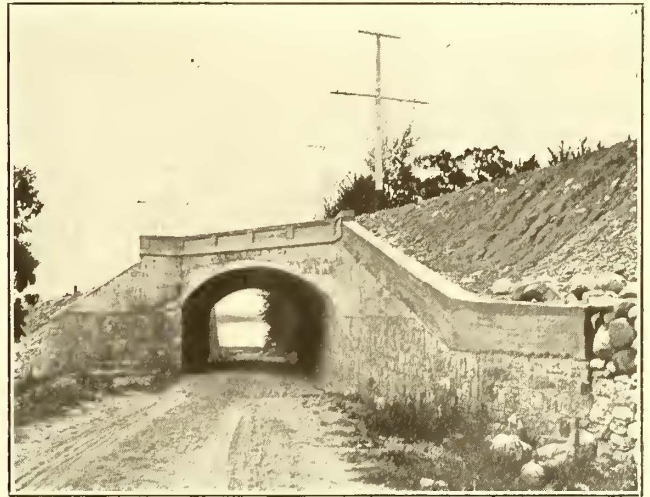
Milwaukee Interurban Lines—Grade Separation on Waukesha Line
