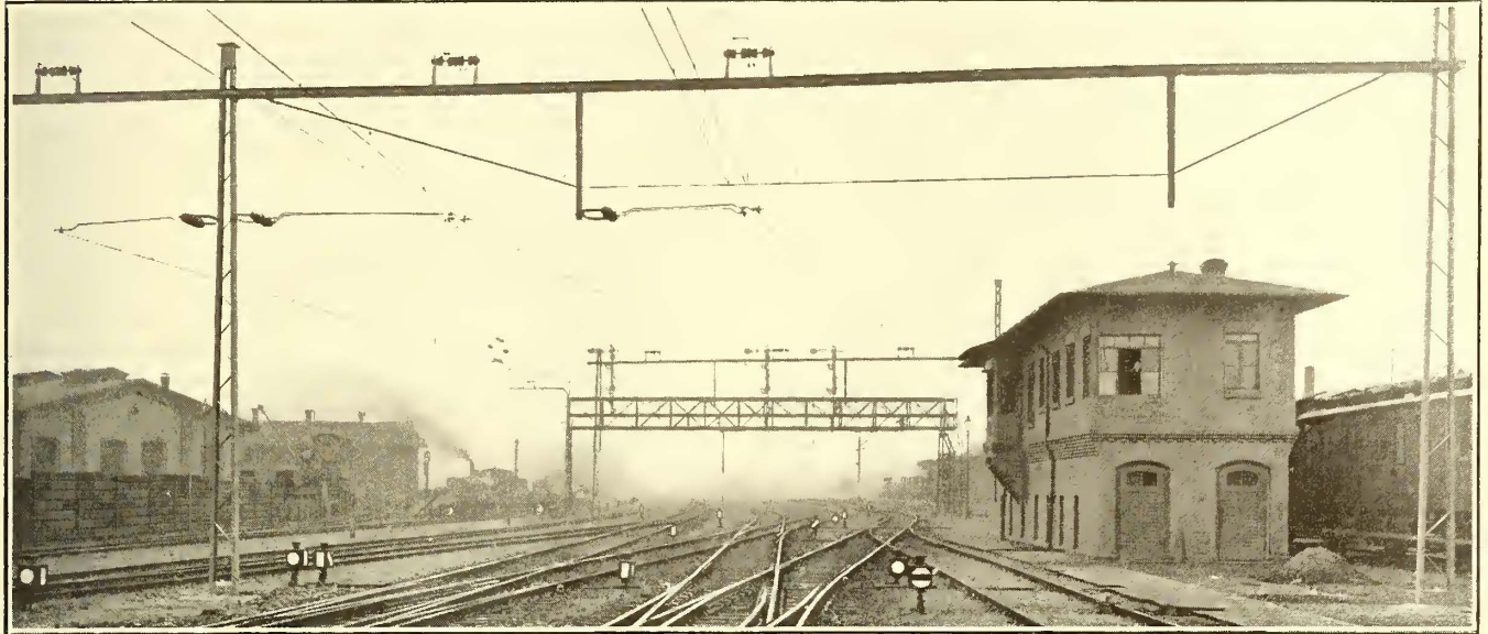
Dessau-Bitterfeld Electric Railway—Catenary Bridge Over a Curve, with Signal Bridge in the Background
