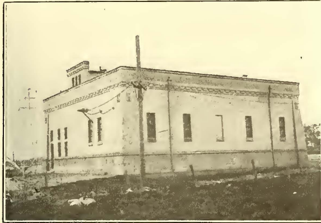
Milwaukee Interurban Lines—Waukesha Beach 1200-Volt Substation Building
