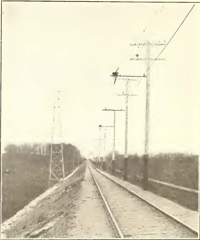
Milwaukee Interurban Lines—Dead Section Between High and Low Voltage Lines
