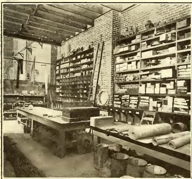
Denver Power—Storeroom in Power Station
