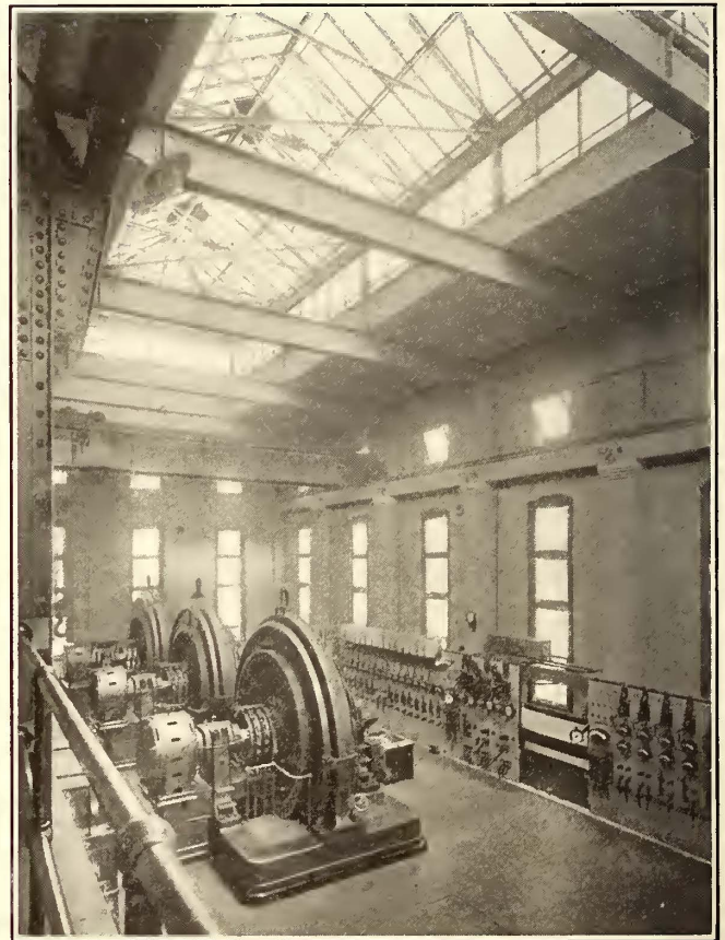
Brooklyn Substation—Monitor Roof and Side Windows as Seen from the Gallery
