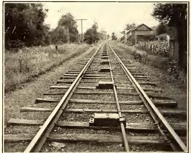
Contact Boxes in Straight Track
