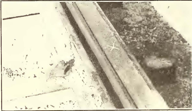
Romapac Rail—Cross Showing Joint of Head Rail After Being Crimped
