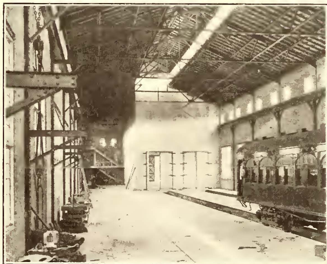
Joliet Extension—Interior of Repair Shop
