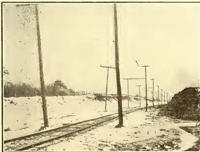
Joliet Extension—Span Wire Catenary Construction
