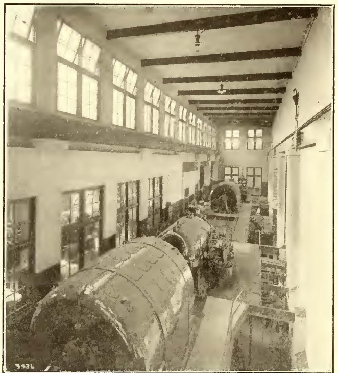
Utah Light & Power—General View of Turbine Room Showing New 8500-kw Turbine
