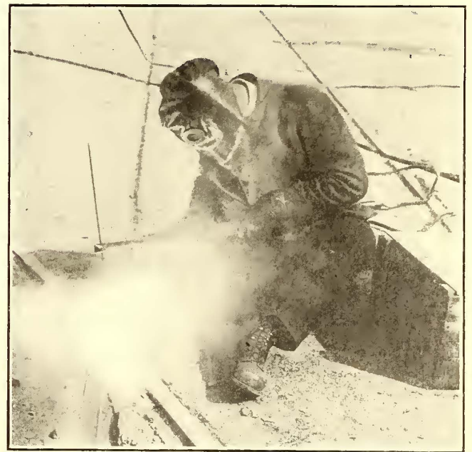
Electric Arc Welding—View Showing Apparatus in Use on Track Work
