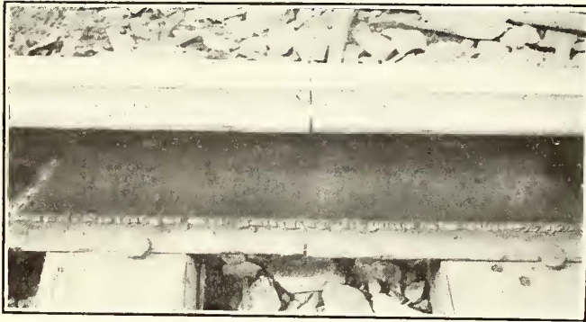
Electric Arc Welding—Welded Fishplate Which Eliminates Necessity for Bonds
