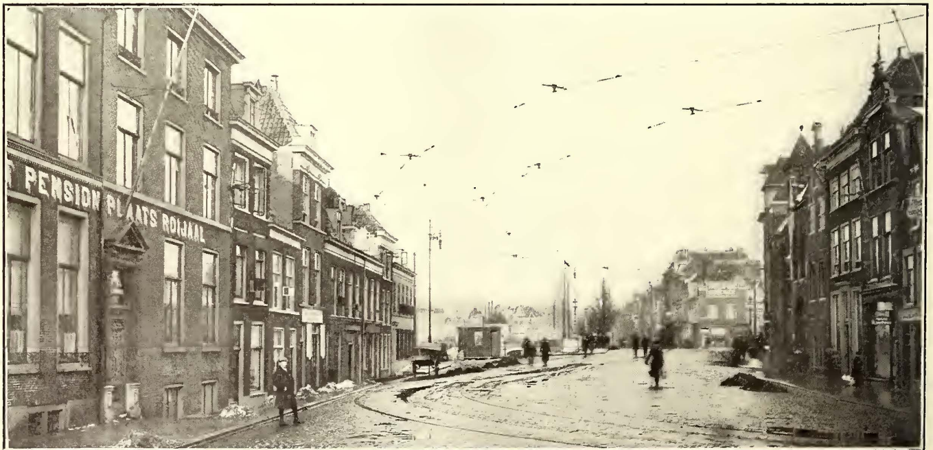
Leyden-Katwyk-Noordwyk Railway—Span Suspension on a Curve in Leyden, Showing Also the Protective By-Pass for Trolley Wire at the Hanger
