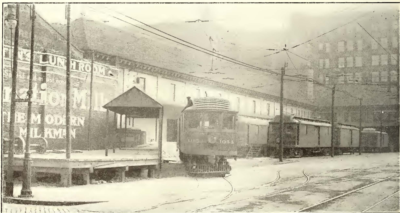
St. Louis Freight Terminal—View Showing Entrance to Freight House Tracks and Milk Platform
