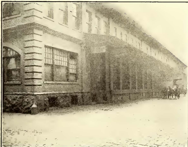
St. Louis Freight Terminal—View of Team Side of Freight House
