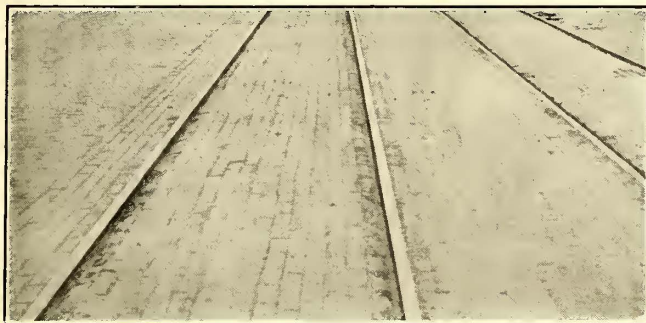
Lexington Track—View of Standard Pavement Between T-Rails
