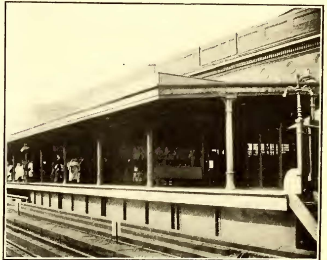
Boston Improvements—Southbound Train Platform, Sullivan Square Terminal
