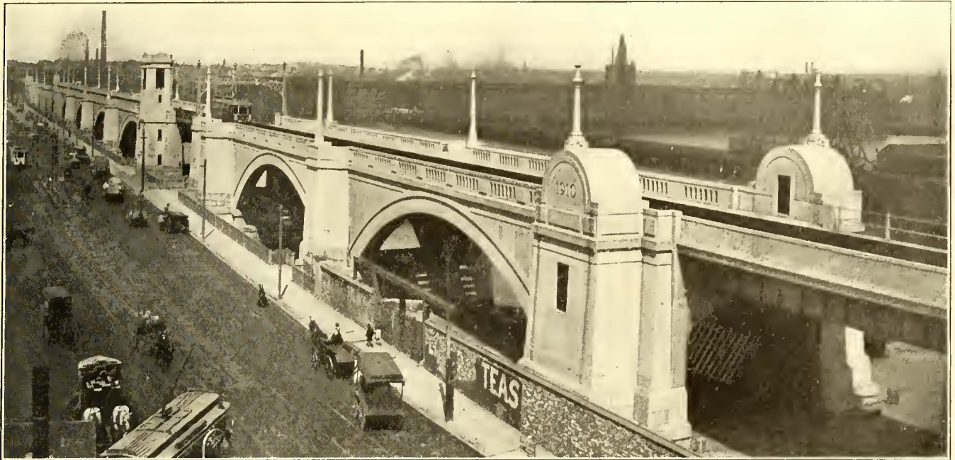
Boston Improvements—General View of Viaduct on the East Cambridge Extension
