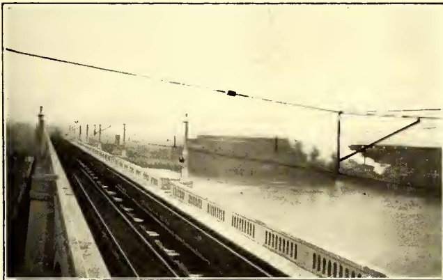
Boston Improvements—East Cambridge Viaduct Extension from Drawtender's Tower
