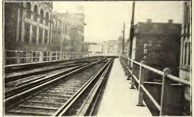
Boston Improvements—Elevated Extension for Viaduct Cars, Causeway Street
