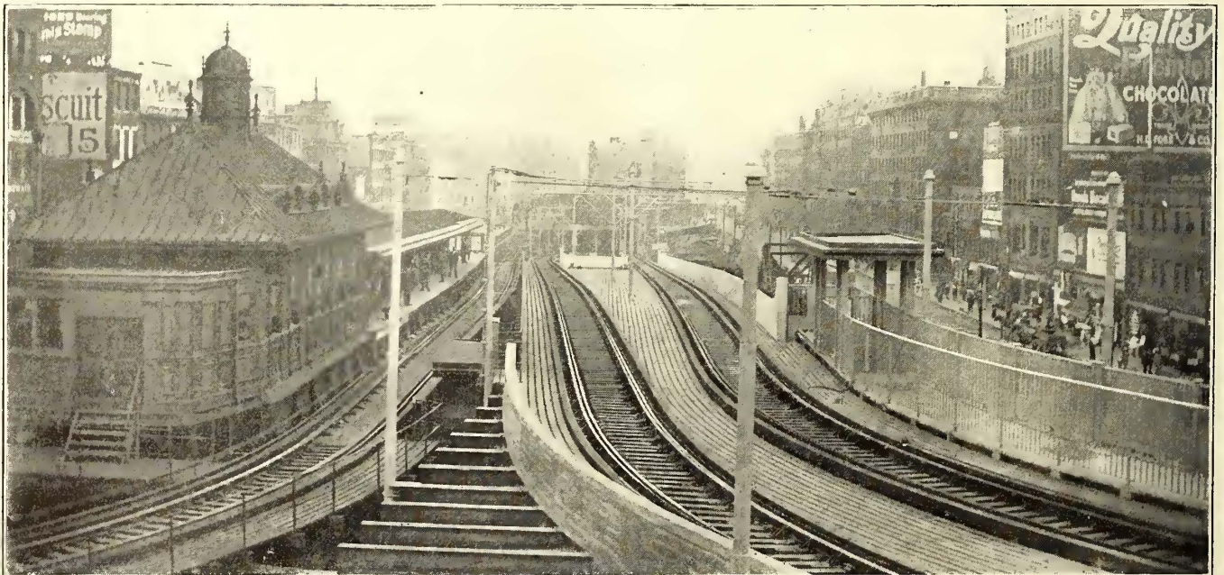
Boston Improvements—North Station Incline, Showing Southbound Tunnel Train Tracks and East Cambridge Viaduct Car, Northbound and Southbound Tracks and Foot Passage
