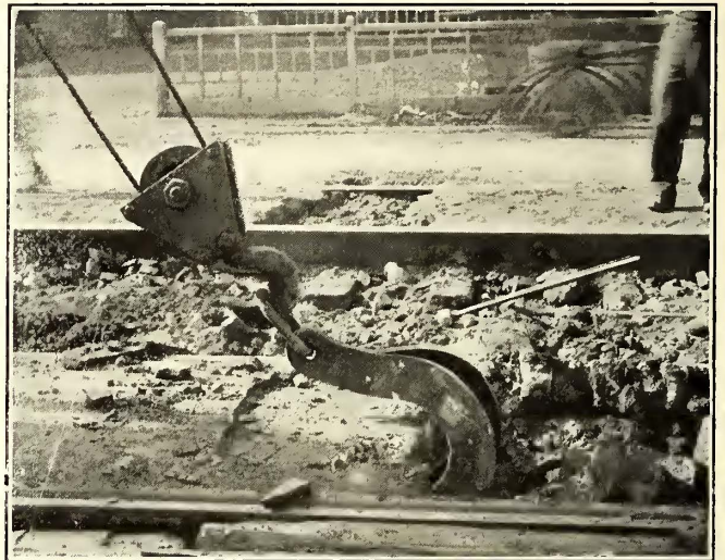
San Francisco Track—Pronged Hook for Tearing Up Concrete
