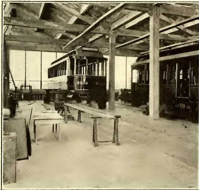
Norfolk Installation—Painting Section of Reinforced Concrete Shop
