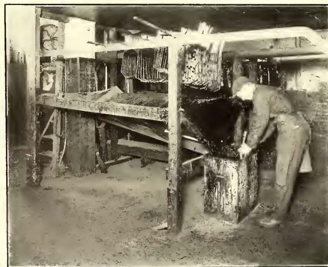
B. R. T. Electrical Shops—Dipping and Hanging Coils
