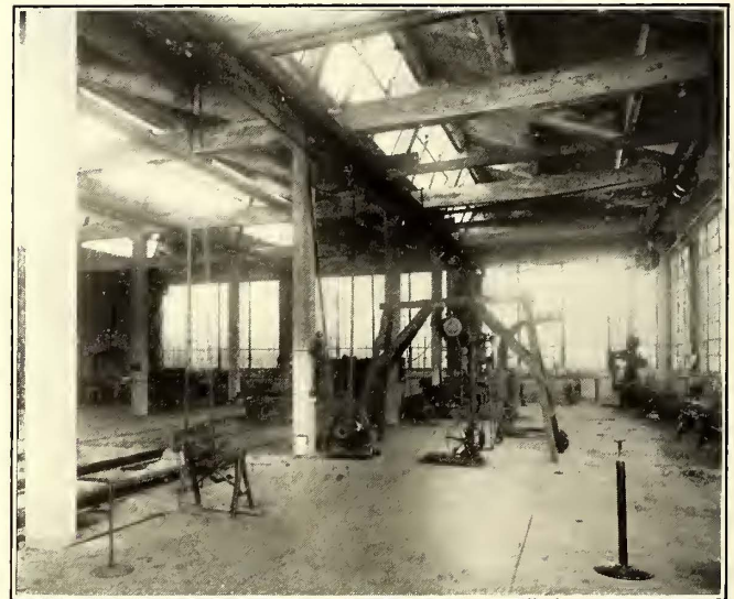
Norfolk Installation—Roof, End and Side Lighting in the Machine Room
