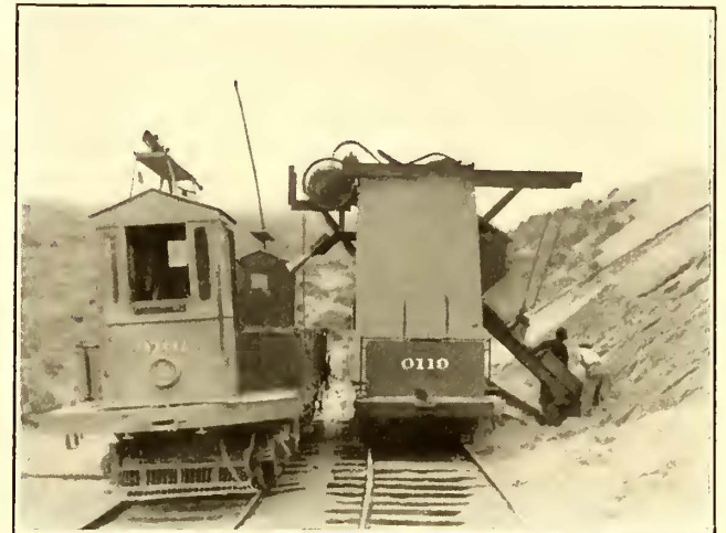
San Francisco Track—Sand Elevator in Operation Loading a Supply Car
