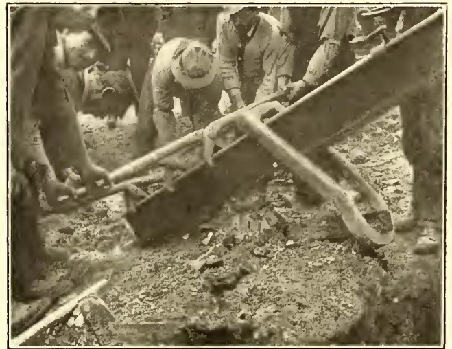
San Francisco Track—Portion of Lever and Link Over End of Cable Yoke
