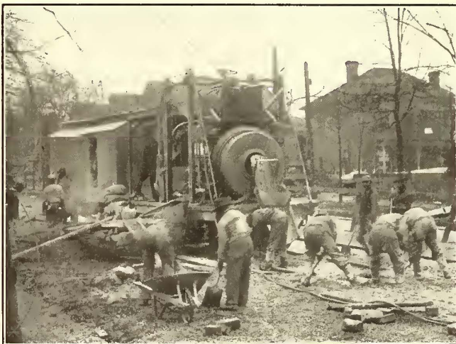
Concrete Mixer for Track Work at Birmingham
