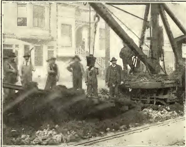
San Francisco Track—Pulling Old Electric Track with Derrick
