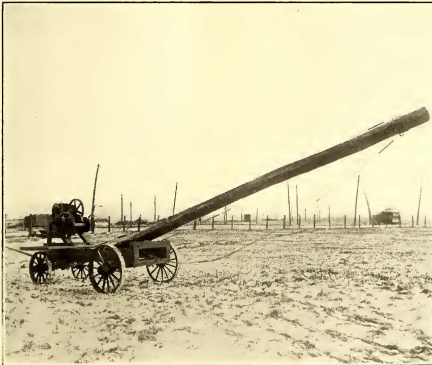
Concrete Poles in Syracuse—Views of Derrick Wagon Used for Installing Poles
