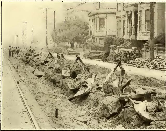
San Francisco Track—Dismembered Cable Track Ready for Excavator
