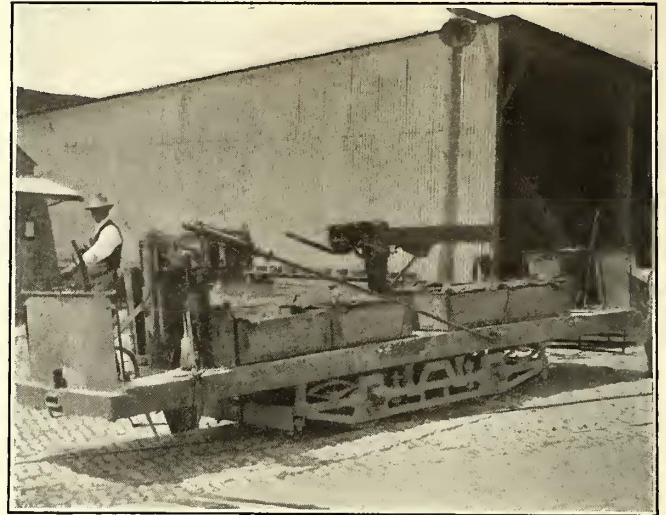
San Francisco Track—Bitumen Car with Trolley Pole Collapsed and Crane Made Horizontal
