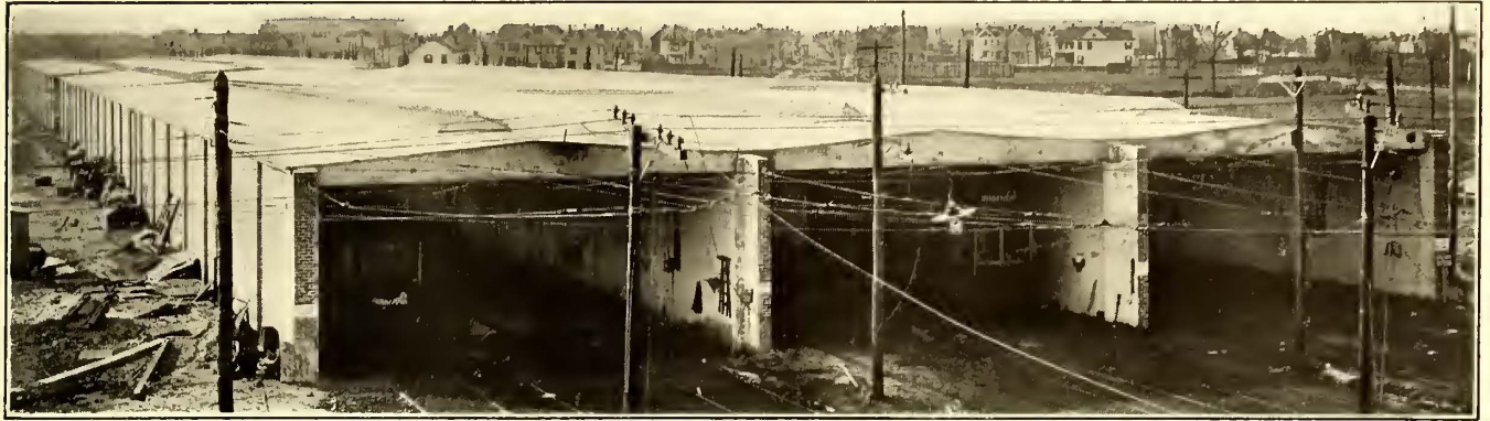
Norfolk Installation—General View of One of the Three-Bay Carhouses, Showing the Unusual but Most Economical Form of Roof and Most Favorable Skylight Arrangement
