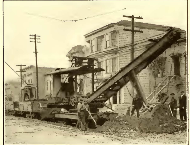
San Francisco Track—Excavating Trench for Track with Shovel Car
