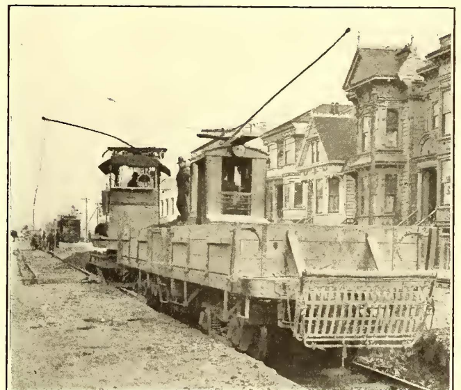
San Francisco Track—Shovel Car in Service Laying Its Own Tracks
