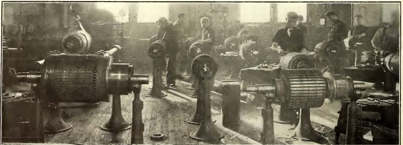
B. R. T. Electrical Shops—Part of Fifty-second Street Shops, Showing Armature Workstands, Armature Sling Carried from Crane Track, Hydraulic Press, etc.
