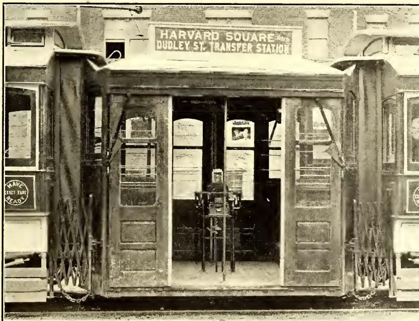
Improved Articulated Car—View of Central Section Showing Roller Curtains and Hinged Hoods—View of Interior Showing Heater Under Step at Right
