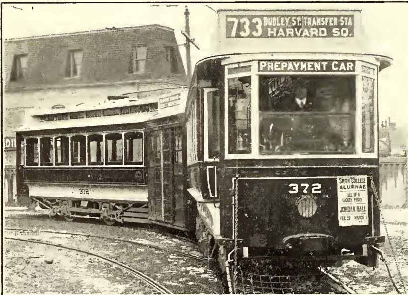
Improved Articulated Car—Car on Curve—Central Section with Outside Folding Doors in Closed Position
