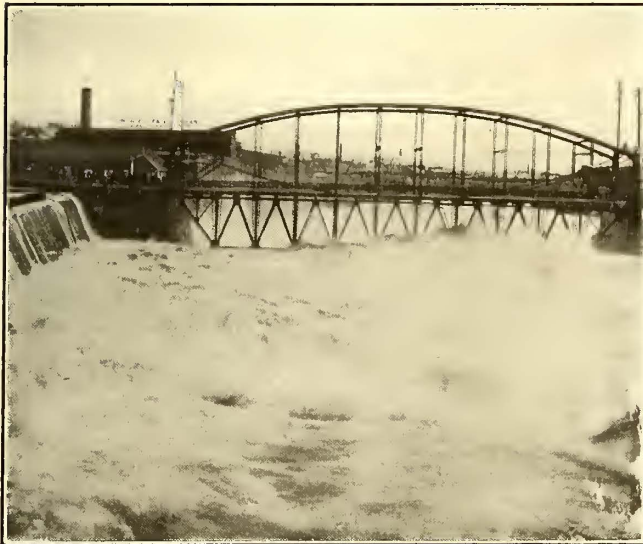
Flood Disaster—Hudson River at Glens Falls, N. Y., Showing Bridge Before Its Collapse
