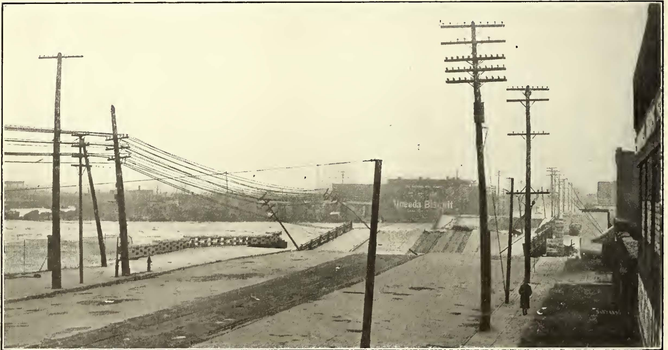
Flood Disaster—Washington Street Bridge in Indianapolis After Its Collapse
