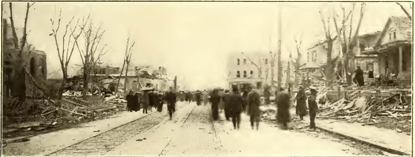
Omaha Tornado—View on Street Showing Complete Disappearance of Trolley Wire and Trolley Poles
