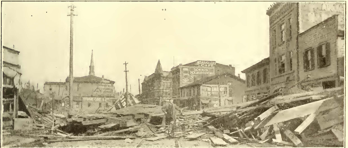
Flood Disaster—Debris Covering the Street Railway Tracks in Dayton, Ohio
