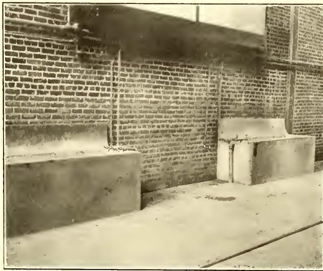
Detroit Paint Shop—Concrete Vats for Washing with Hot Water and Lye
