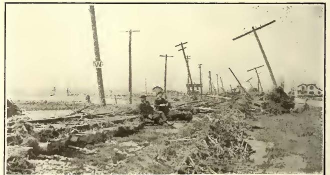
Ohio Flood—Damaged Track Between Springfield and Dayton
