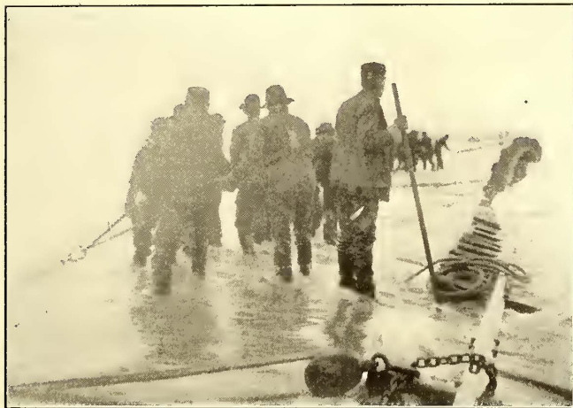
Replacing Railroad Tracks Overturned by the Flood
