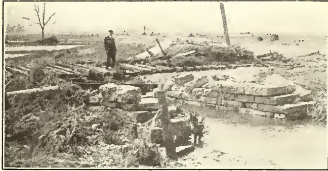
Ohio Flood—Washed-Out Culvert on Ohio Electric Railway
