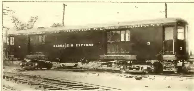
Express Car for Automobiles—Side View, Showing Wide Side Doors
