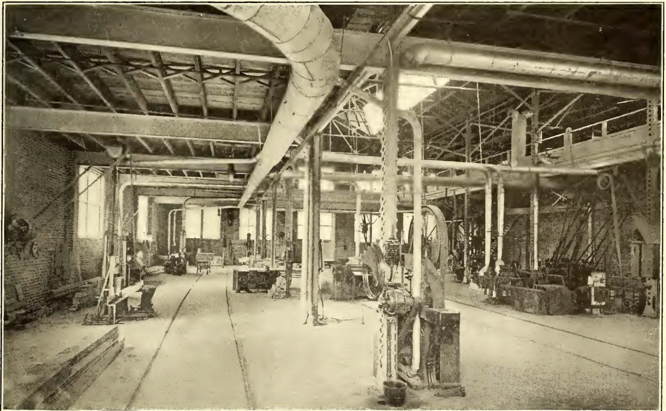
Omaha Wood Shop—Interior View of Wood Mill from First Floor, Showing Balconies Along Both Sides
