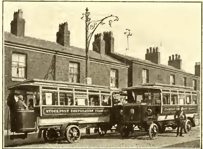
Stockport Trackless Trolley—Opposing Cars Interchanging Current Collectors
