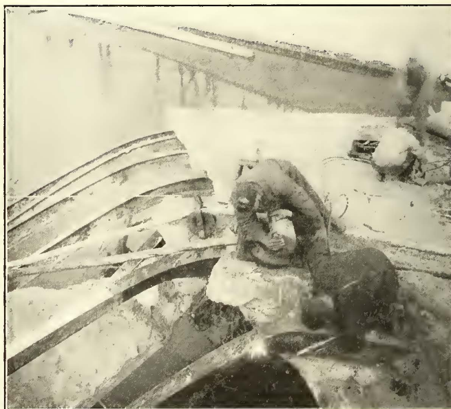
Cutting Away Floor Beams of Wrecked Bridge with Oxy-Acetylene Flame
