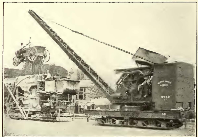
Handling Concrete Aggregate in Wagon Loads at Detroit
