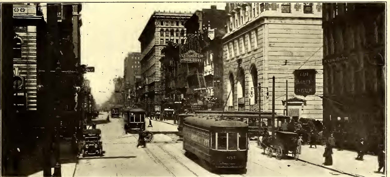
Buffalo Car Maintenance—View at Most Congested Point in the City, Showing New and Old Types of Car
