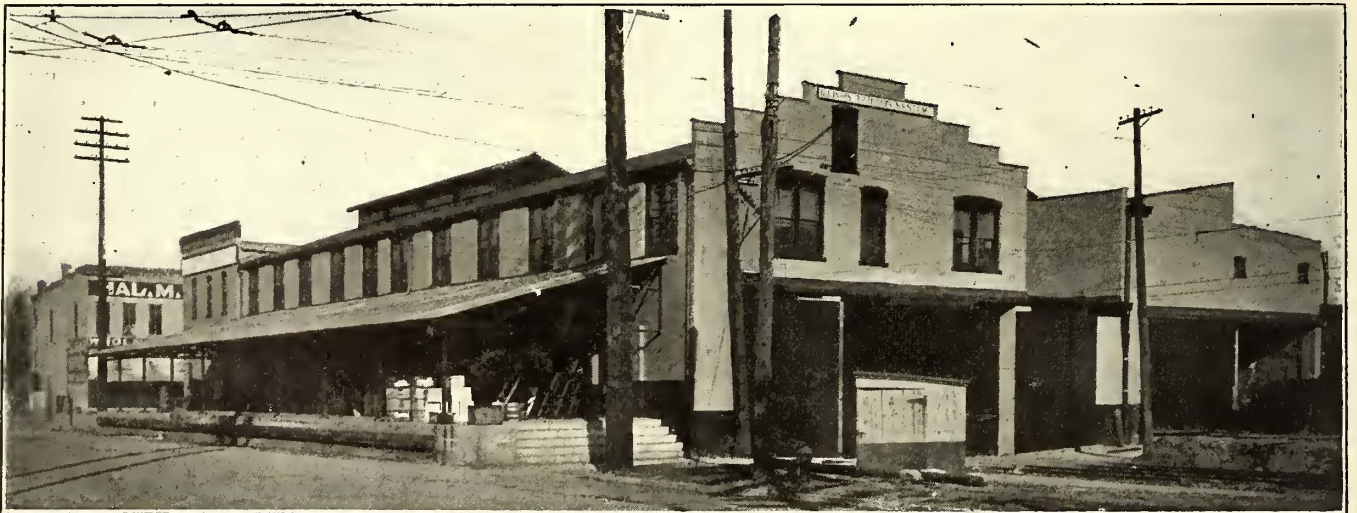
Springfield Freight House—View Showing Entrance Doorways and Receiving Platform
