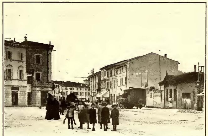
Verona-Caldiero 1300-Volt D. C. Railway—Construction on City Streets
