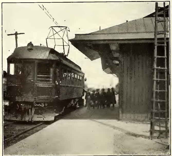
Erie Electrification—Standard Car at Avon Station
