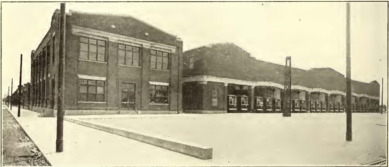
Luzerne Carhouse—Rear View, Showing Transportation Building at Left, Sand-Handling Bay Across the Rear of the Carhouse, Etc.
