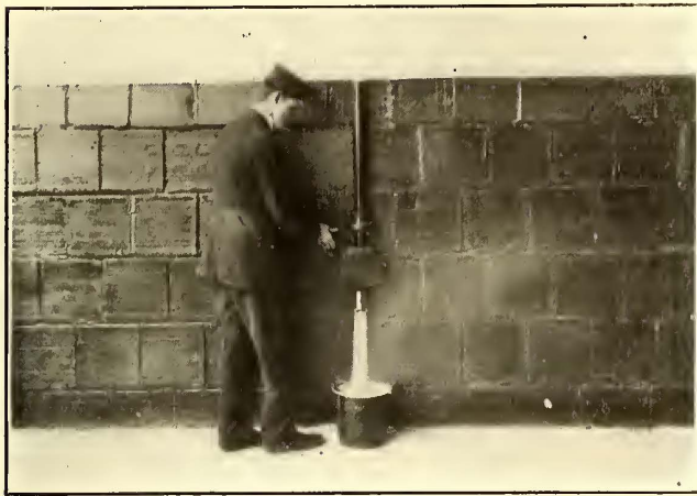
Luzerne Carhouse—Sand Spout Supplied from Storage Bin Above
