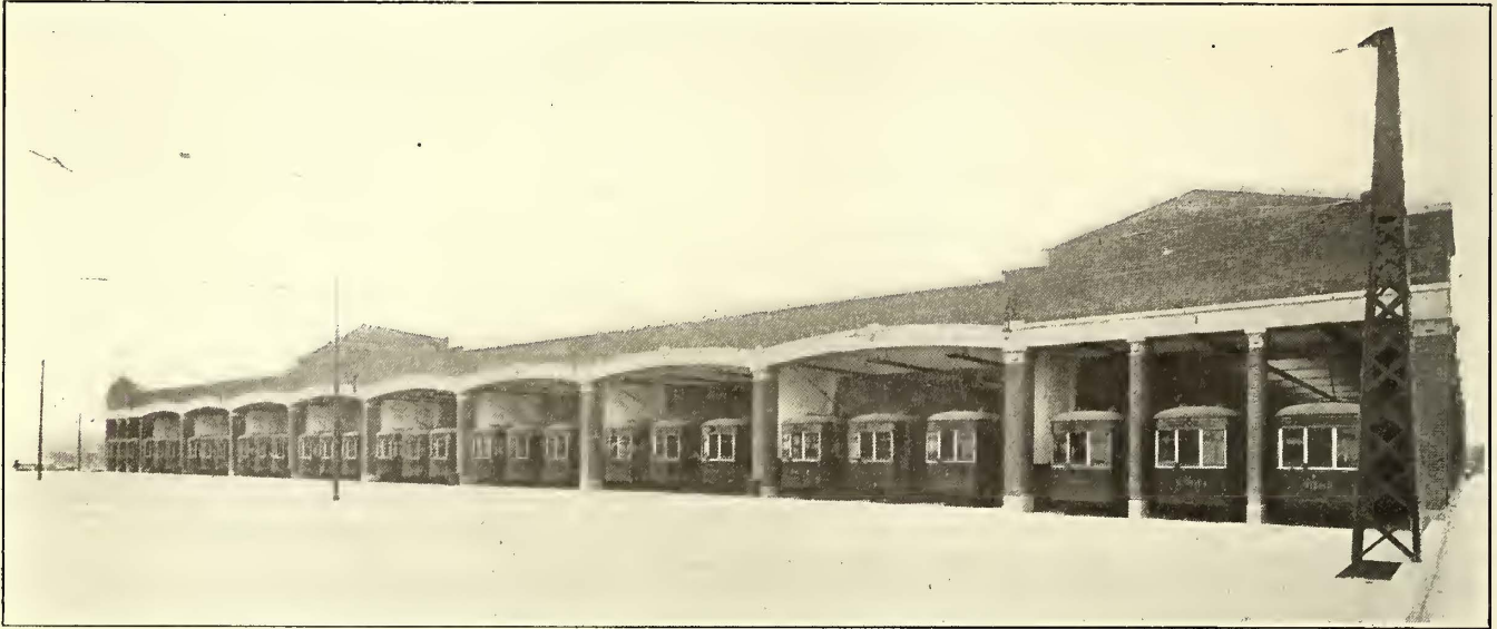
Luzerne Carhouse—Front View, Showing Shop Bay at Right, One of the Catenary Towers, Etc.
