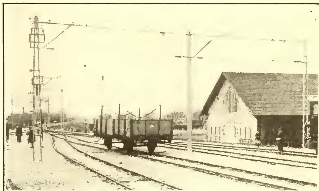
Mittenwald Railway—Light Bridge Construction
