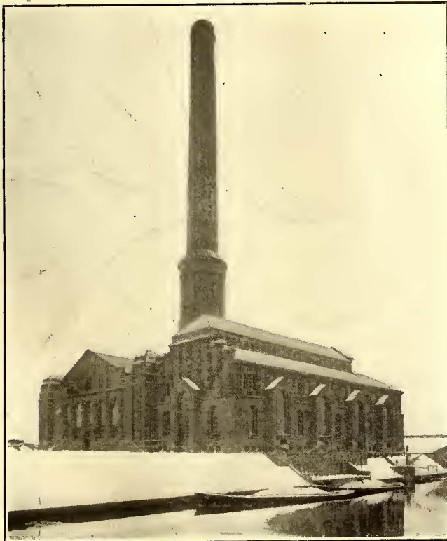
Hamburg Power—Generating Plant at Barmbeck
