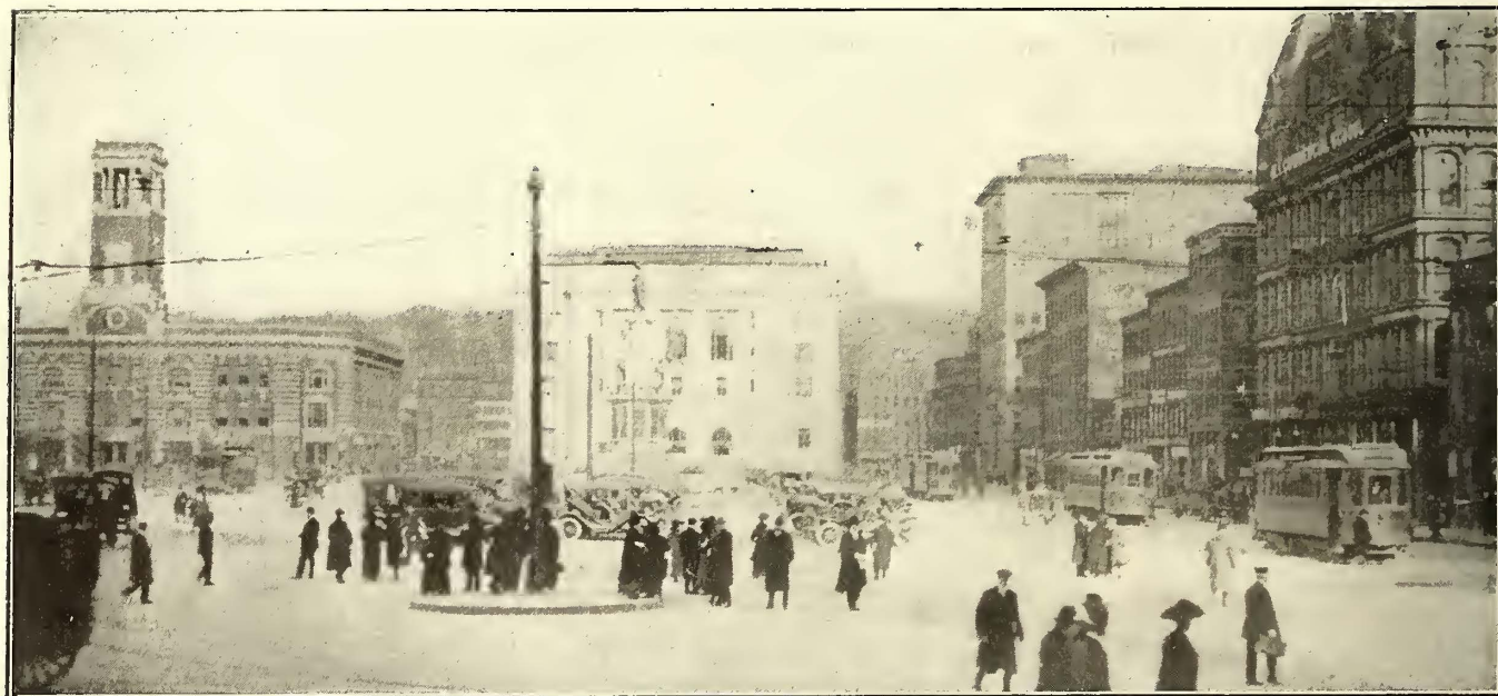
Providence Improvements—Exchange Place Loop
