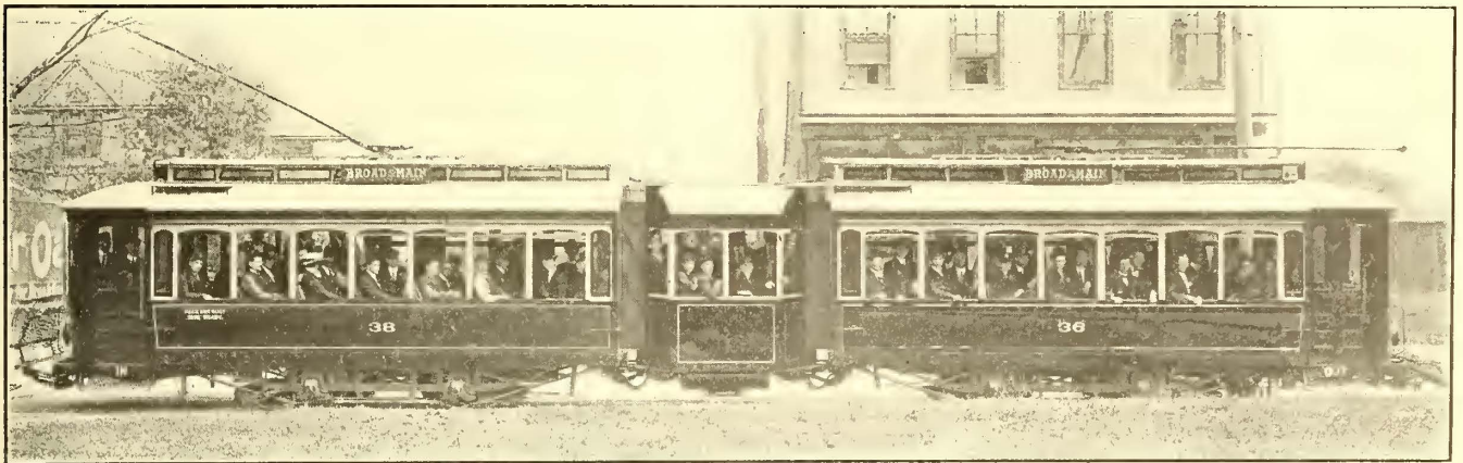
Richmond Articulated Car—General View Showing Arrangement of Car
