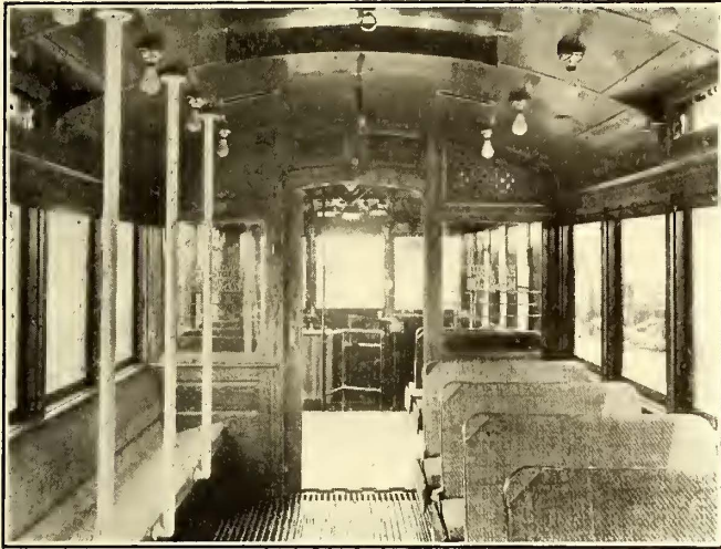
San Francisco Car—Looking from Closed Section Toward Semi-Open Compartment and Platform
