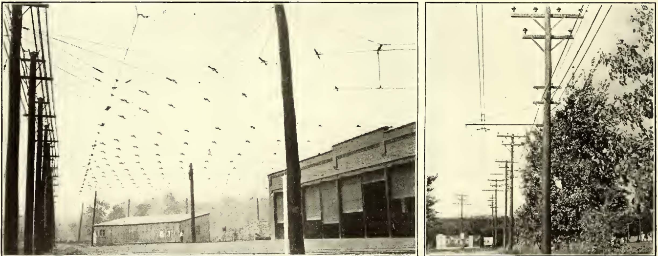
Connecticut Company—Port Chester Carhouse and Typical Trolley Line Construction
