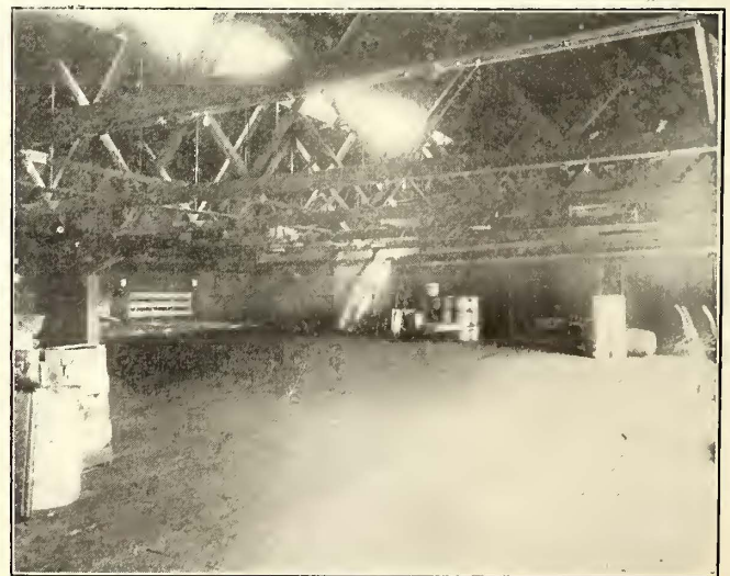
Cops Hill Freight Terminal—Interior
