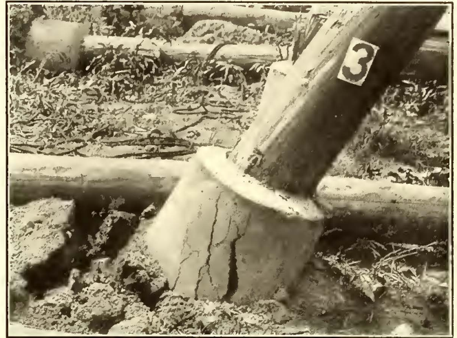
Cracking of Reinforcement Under Excessive Loading
