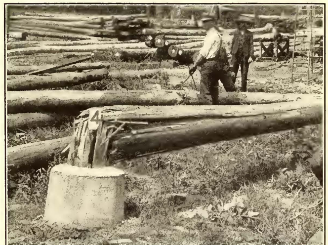
Reinforcement Surviving Breakage of Pole
