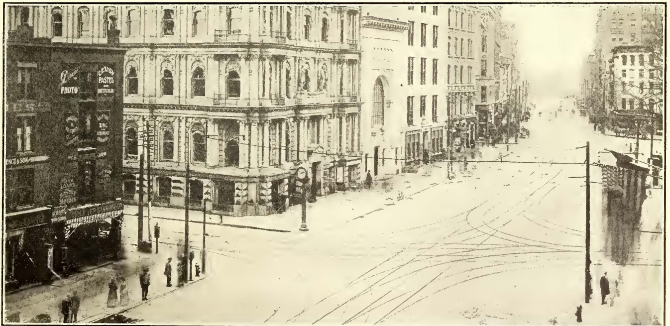
Connecticut Way—View of Completed Special Steel Center Construction at Pearl and Main Streets, Hartford
