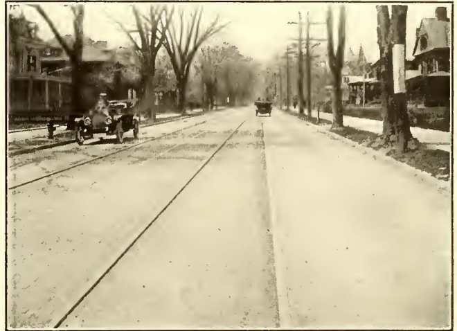
Rail and Paving Results—Four-Year-Old T-Rail in Wood Block on Narrow Street
