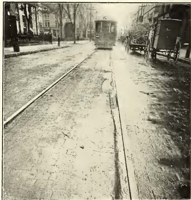
Rail and Paving Results—Hump Block Paving, Bridgeport, After Three and a Half Years' Service
