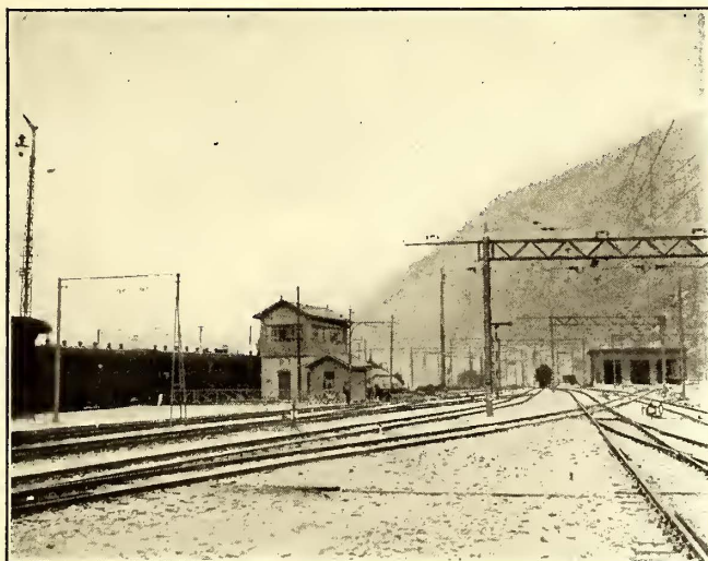
Lötschberg Railway—View of Overhead Construction
