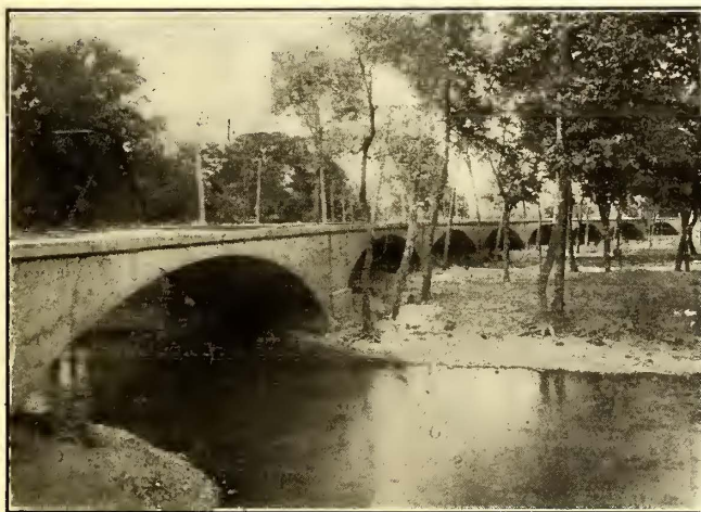
Concrete Viaduct Replacing Wood Trestle and Truss Bridge
