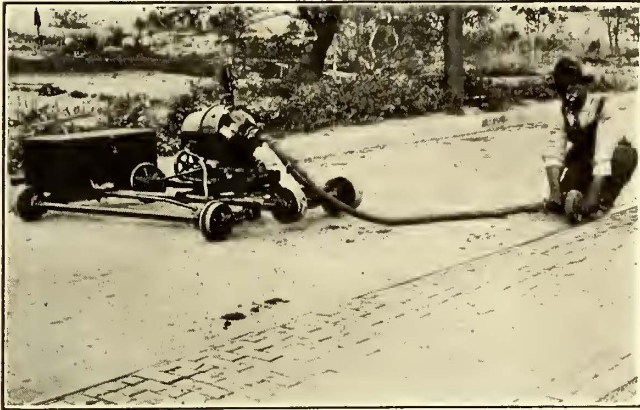
New Rail Grinder—In Position for Hand Grinding
