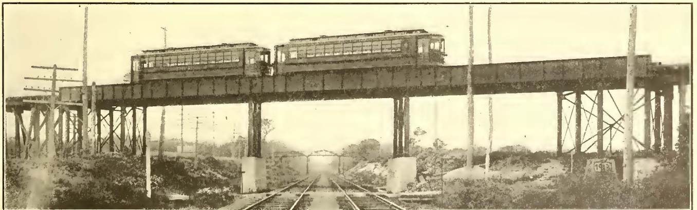
Newark-Trenton Line—Bridge Over Lehigh Valley Railroad Near Metuchen
