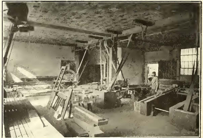
Dayton Carhouse and Shops—Mill Room
