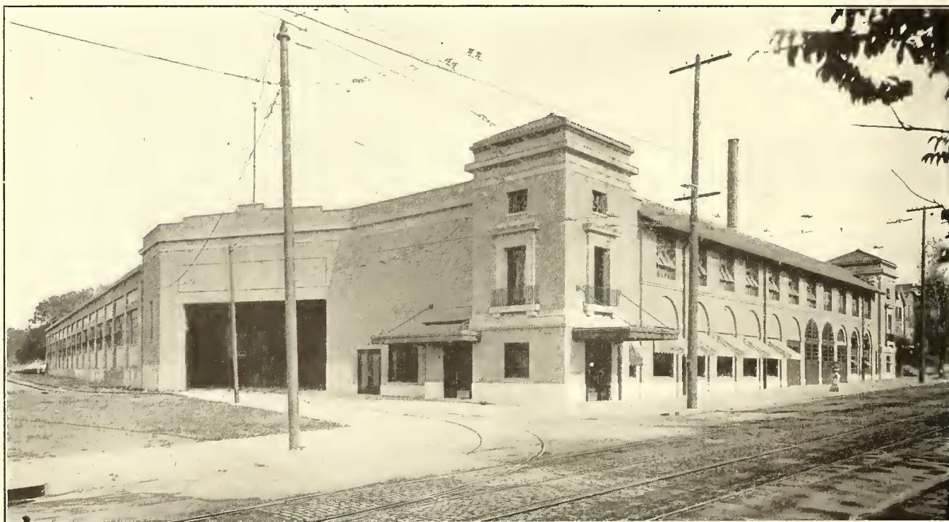
Dayton Carhouse and Shops—General View Showing Office in Front and Entrance for Cars at Side
