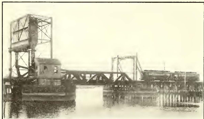
Newark-Trenton Line—Bascule Drawbridge Over Rahway River
