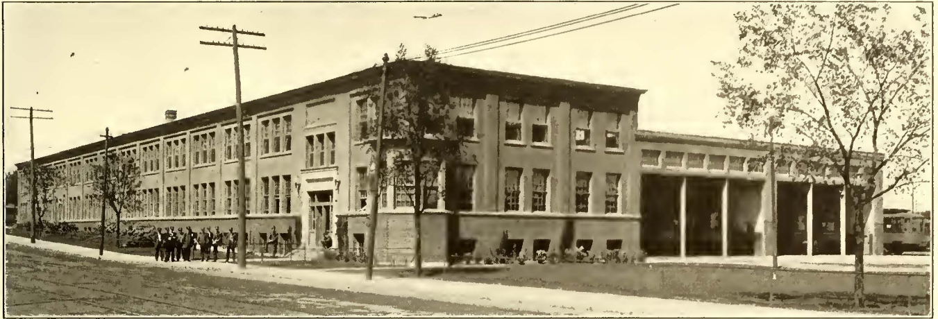
Twin City Welfare Work—Lake Street Carhouse
