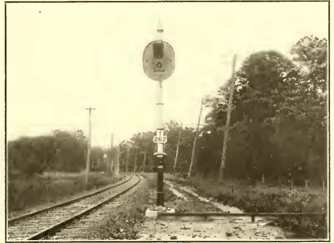
Newark-Trenton Line—Type of Intermediate Signal on the New Right-of-Way Division
