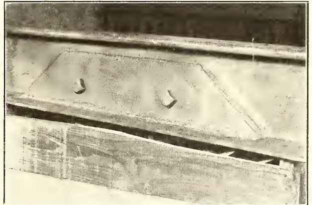
Electrically Welded Rail Joint, Pacific Electric Railway, Los Angeles
