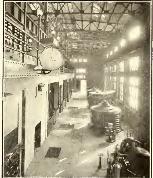
Views of 10,000-kw Generator and of Interior of Las Plumas Hydroelectric Station, Great Western Power Company
