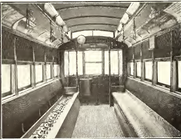
Storage Batteries Under Longitudinal Seats, Third Avenue Railway
