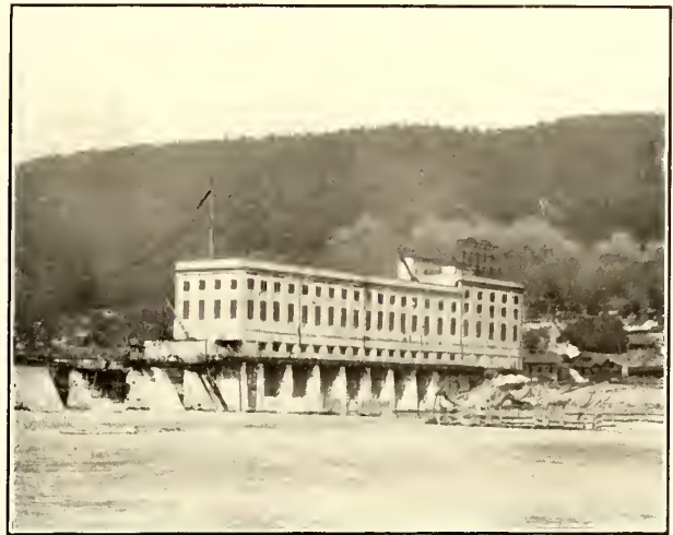
Power House and Part of Dam, Hale's Bar Hydroelectric Station
