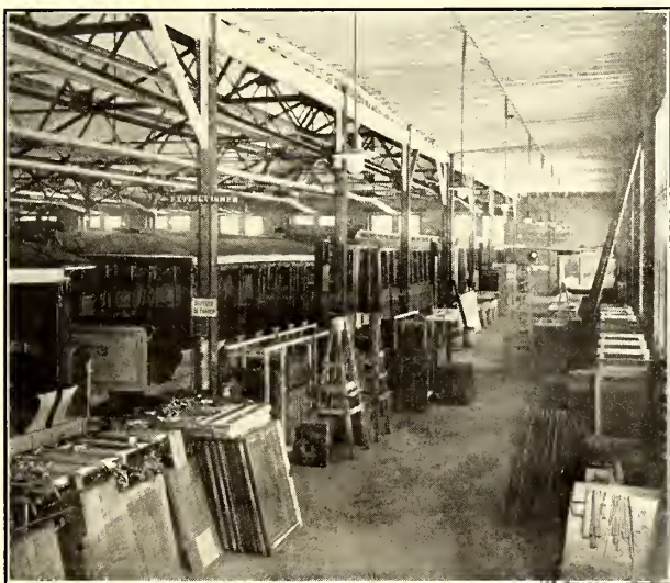
Sash Room at End of Paint Shop, Montreal Tramways
