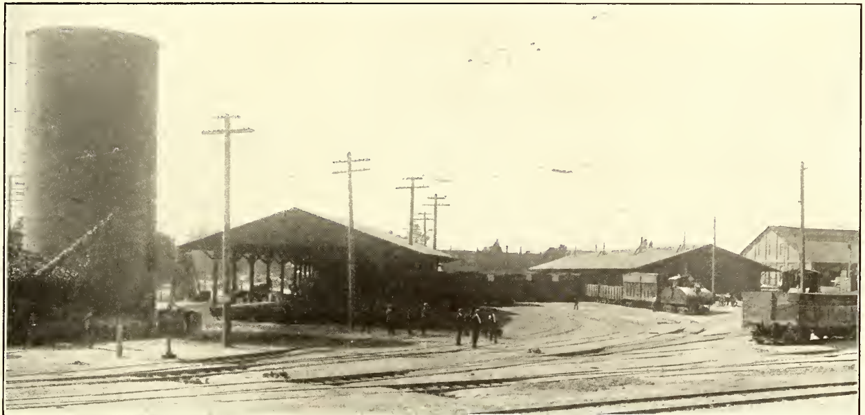
Freight Depot and Tracks at Los Angeles, Pacific Electric Railway—Receiving Shed at Left and Delivery Shed at Right
