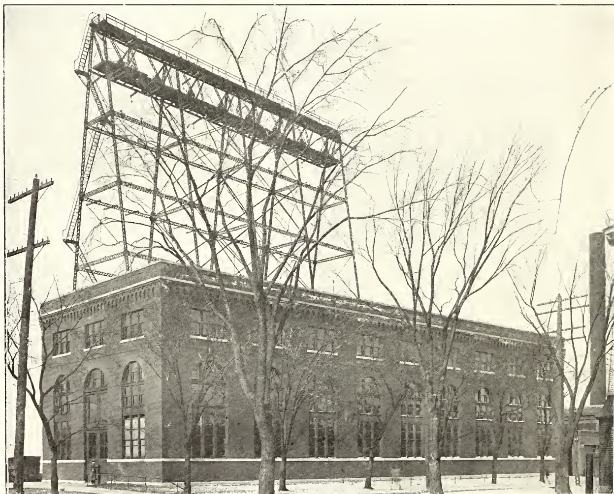
Terminal House of Cataract Power & Conduit Company with Tower for 1700-ft. Span Across Niagara River
