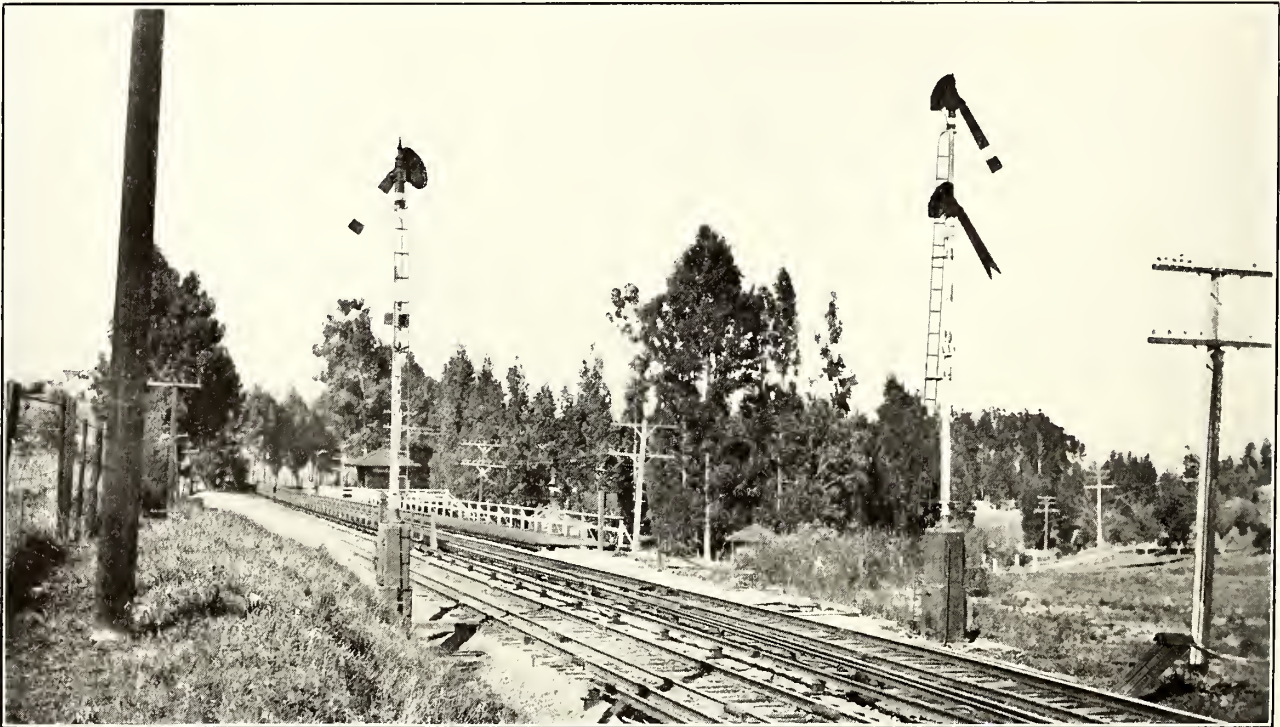
View on Northwestern Pacific Railroad, the First Line to Be Equipped with A. C. Signals, Showing Home and Distant Blades on One Mast Because of Short Block in Advance
