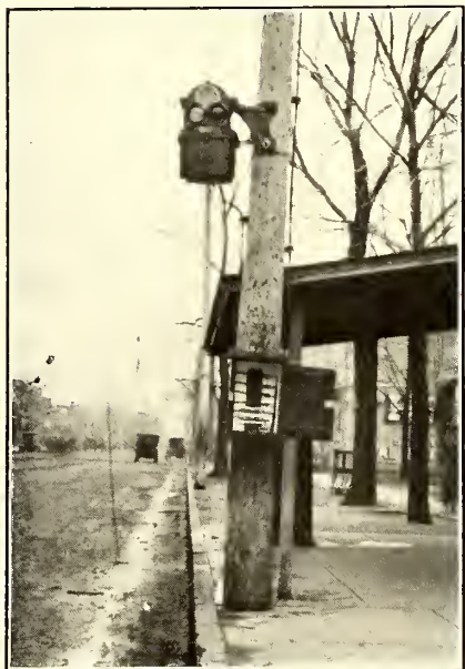
Trolley-Contact Signal for Interurban Service in South Bend, Ind.
