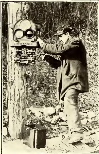
Making Repairs to Trolley-Contact Signal in the Field
