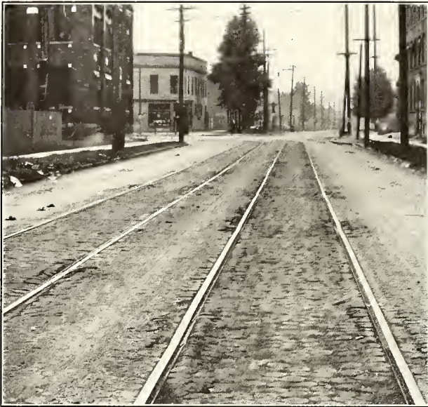
Detroit United Railway—Old-Style Maintenance with Joints Cupped and Paving Disturbed
