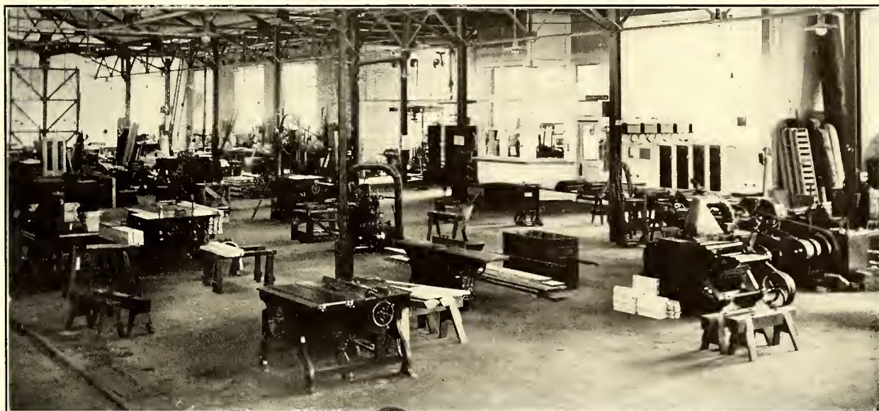
Wood Mill in New Shops of Montreal Tramways, with Concealed Shavings-Exhaust Pipes
