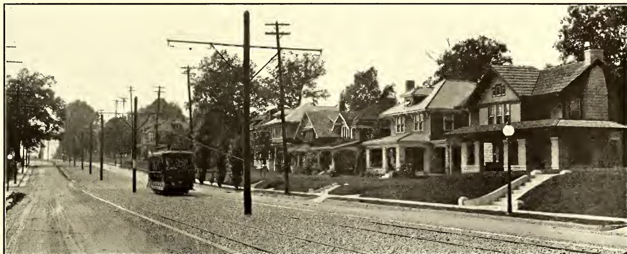
Neutral Strip for Suburban Track Construction, Memphis Street Railway
