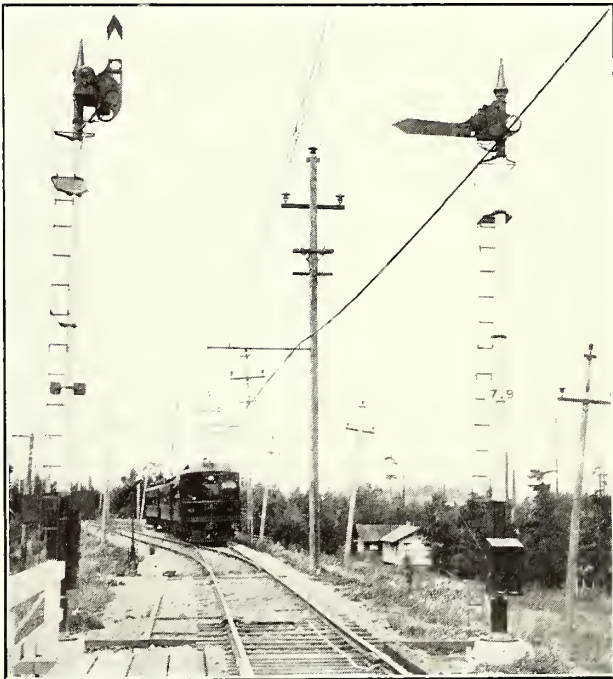
Proceed and Stop Indications with Three-Position Signals, Oregon Electric Railway
