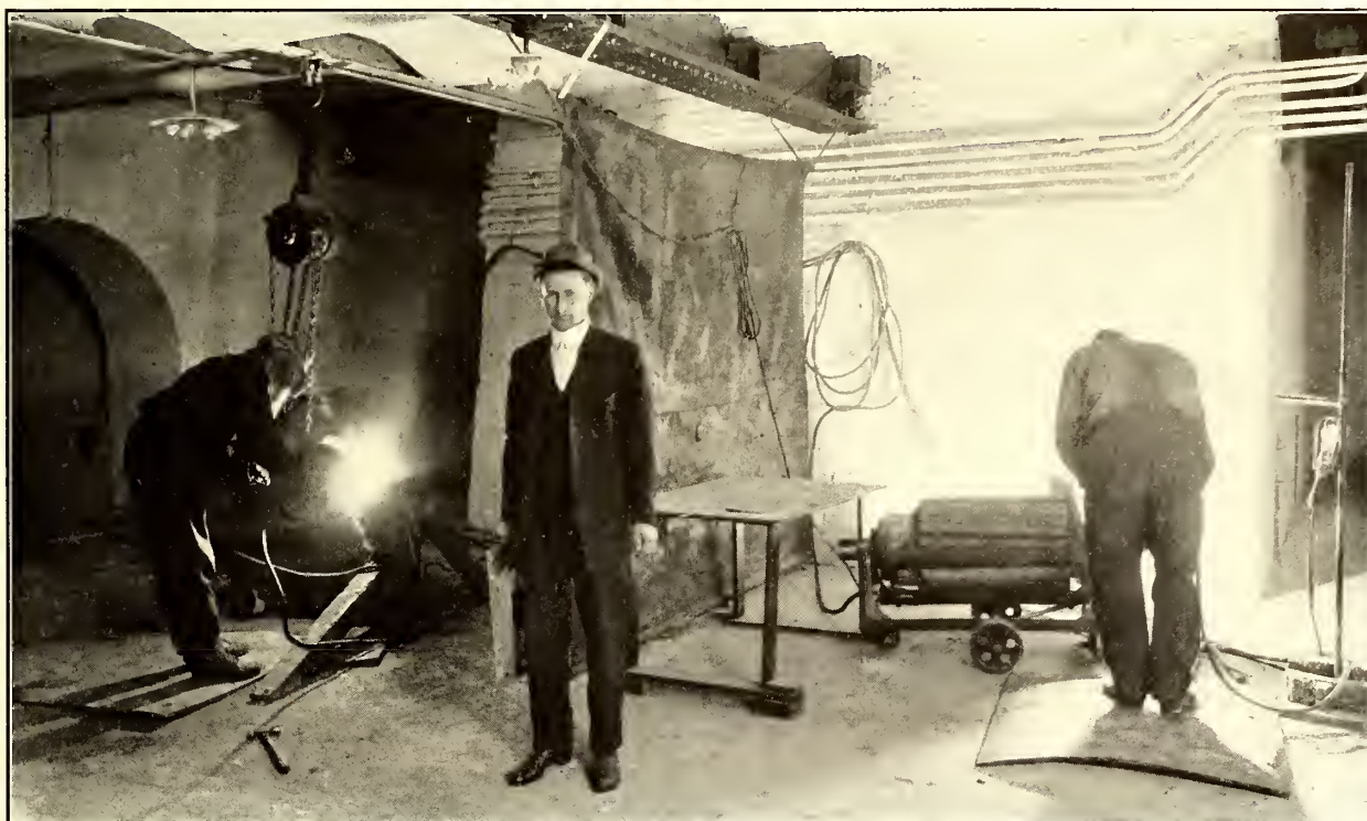
Welding with Electric Arc, Third Avenue Railway, New York
