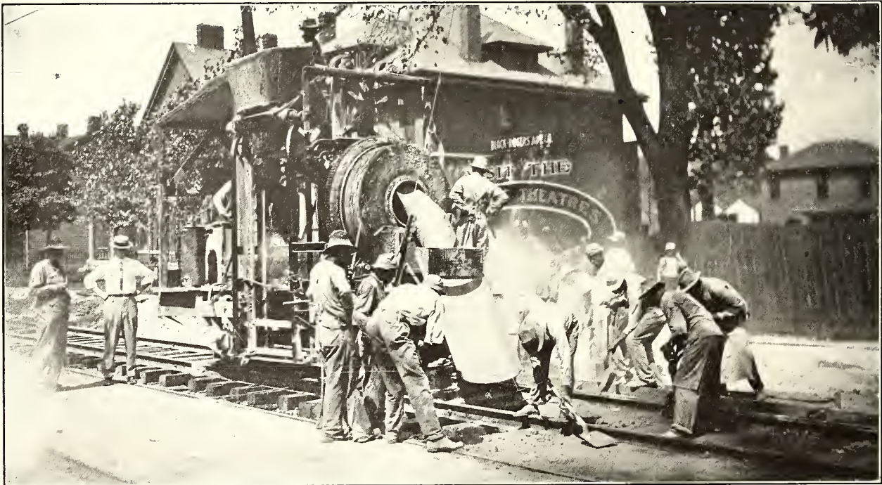
Concrete Mixer Placing Paving Foundation, Memphis Street Railway
