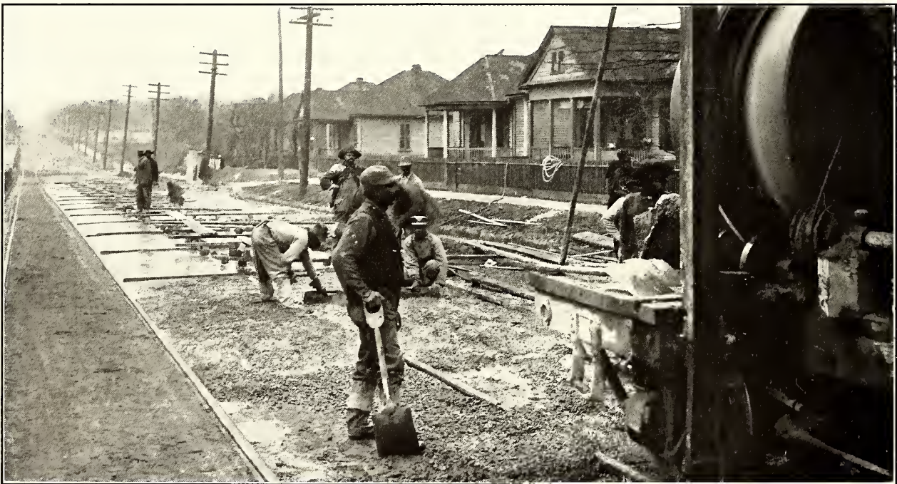
Concrete Paving with T-Rail, Birmingham Railway Light & Power Company
