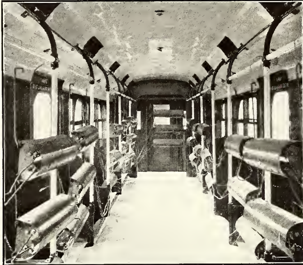
Electric Heaters Hung in Car for Baked Enamel Painting, Hudson & Manhattan Railroad
