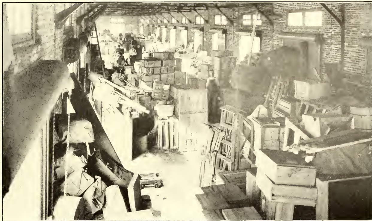
Interior of Dayton Freight House, Ohio Electric Railway
