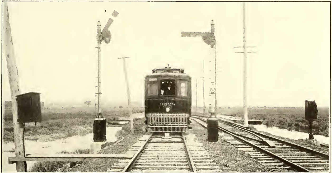
Home Signals for Adjoining Blocks on New High-Speed Line to Trenton, Public Service Railway
