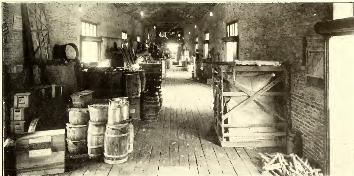
Interior of Joint Freight Station at Indianapolis, Ind.
