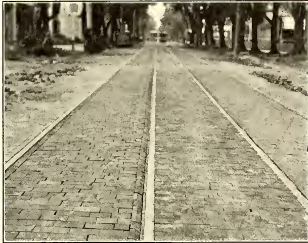
Toledo Railway—View Showing Pavement Before Filling with Sand
