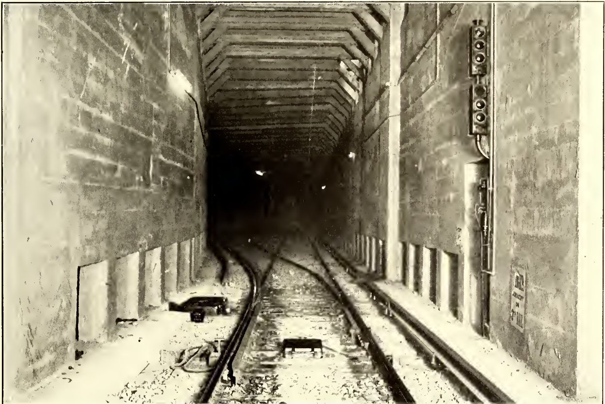
View Showing Three-Indication Signals for Main and Diverging Routes at the Right and Trip for Automatic Stop and Speed Control at the Left, Inter-Bridge Loop, New York Municipal Railways
