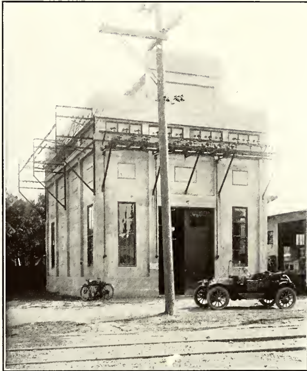
Substation at Sacramento, Great Western Power Company
