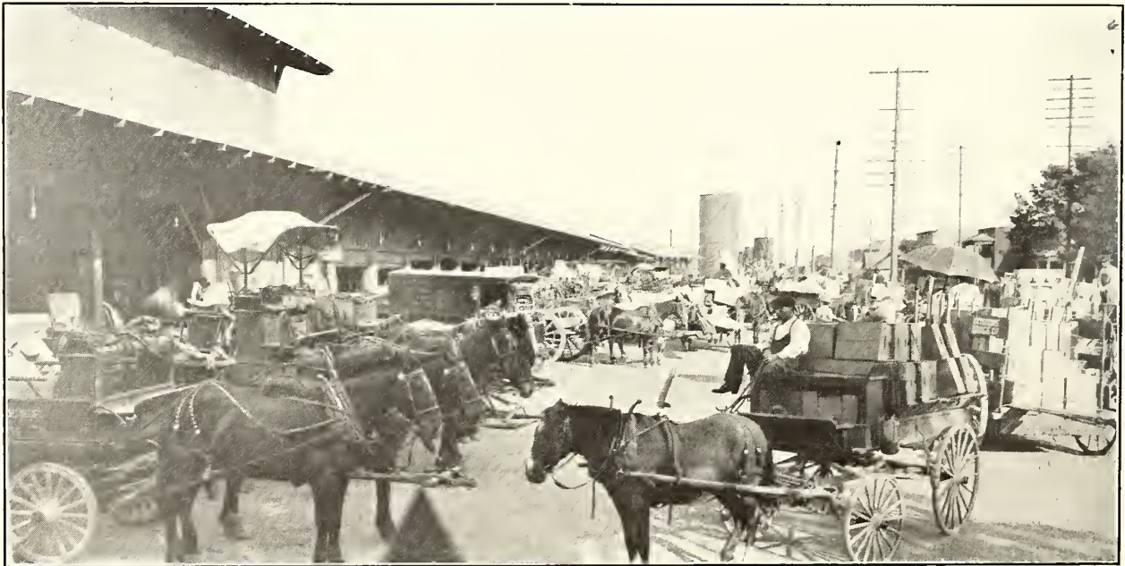
Team Side of Receiving Shed at Los Angeles Freight Terminal, Pacific Electric Railway
