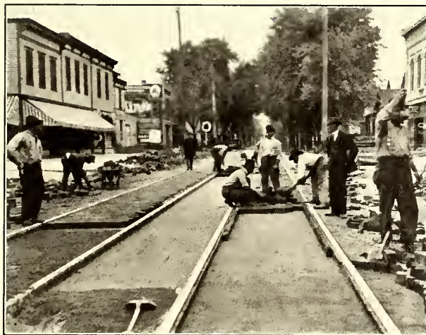
Toledo Railway—Laying Creosote Paving Block on Sand Cushion
