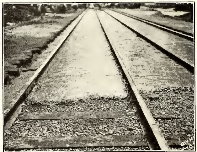
Toledo Railway—Waterproofing Coat of Concrete Laid on Ballast
