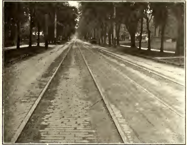
Toledo Railway—View Showing Completed Track and Paving
