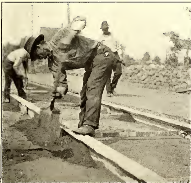
Plastering the Rail Before Paving Is Begun, Chicago City Railway
