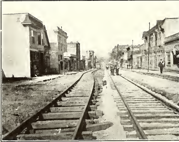
Toledo Railway—New Track Shown Resting on Concrete Foundation and After the Ballast Is Applied
