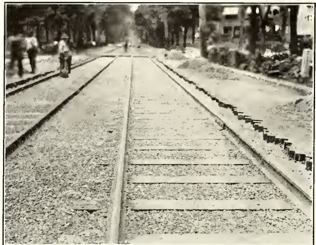
Toledo Railway—Standard Track with Ballast in Place Ready for Paving
