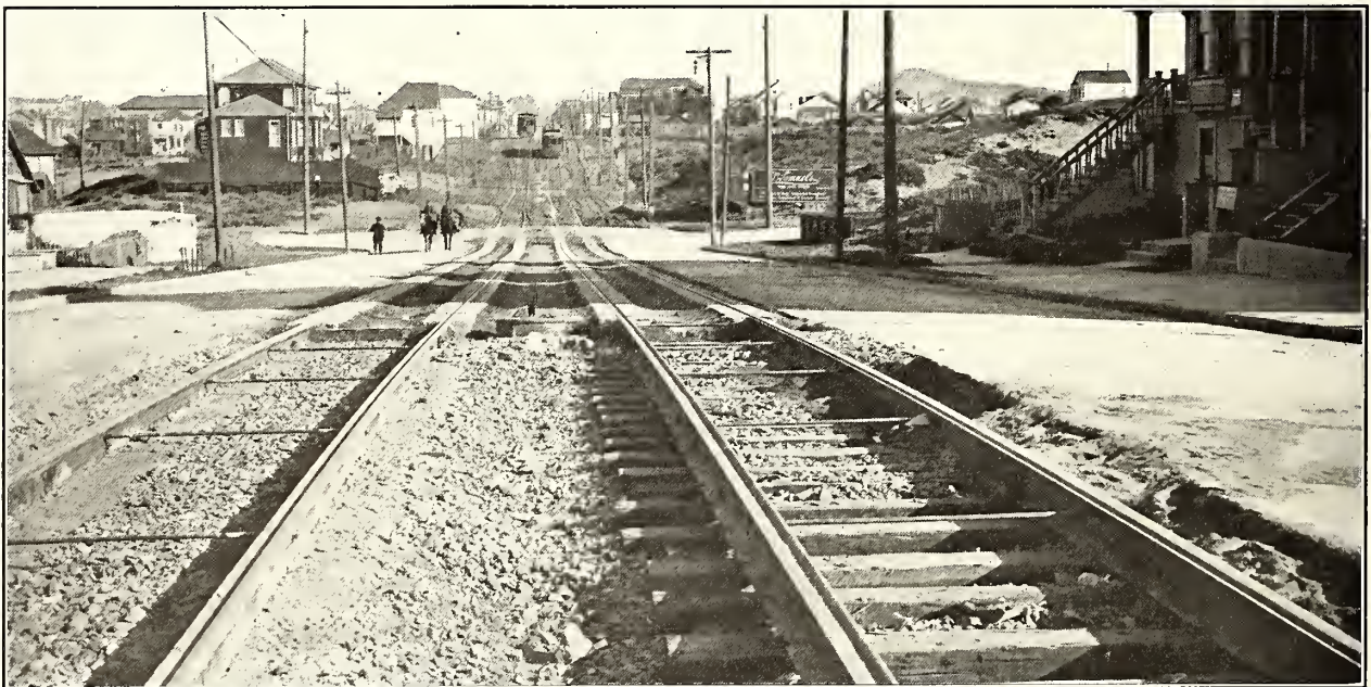
Girder Grooved Rail on Combination Ballast and Concrete Foundation, United Railroads of San Francisco
