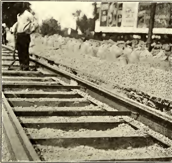
Type No. 3 Track of Chicago City Railway After Tamping Ballast
