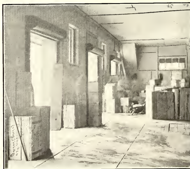
Team-Side Doors, Ohio Electric Freight House at Springfield
