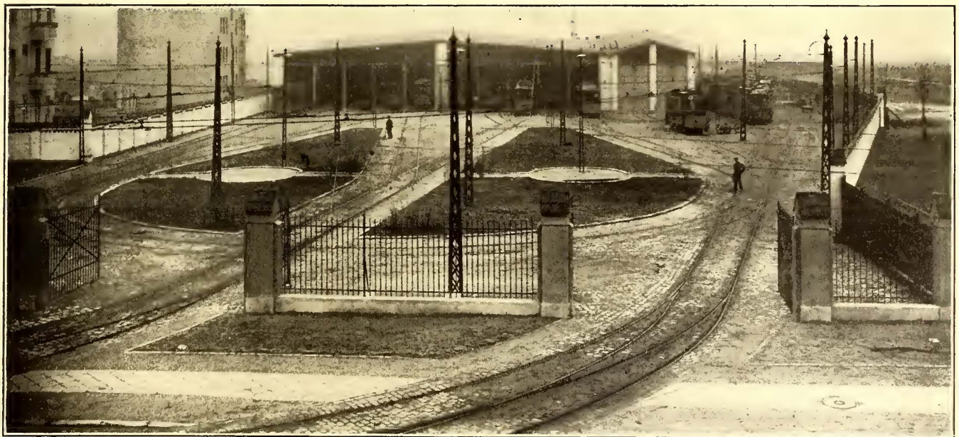
Berlin Carhouses—General View of New Weissensee Carhouse, Showing Switching Yard and Entrance Gates in the Foreground
