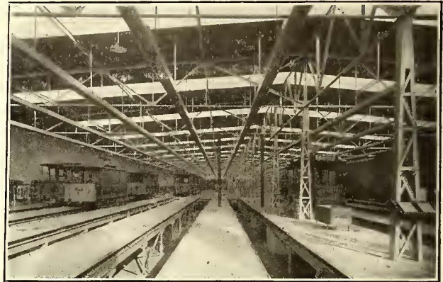
Berlin Carhouses—Interior of New Weissensee Carhouse, Showing Truss Roof and Steel Columns
