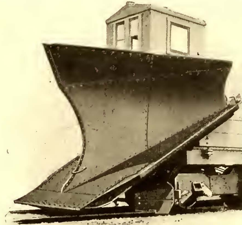
Snow Removal—Combined Snow Plow and Flanger
