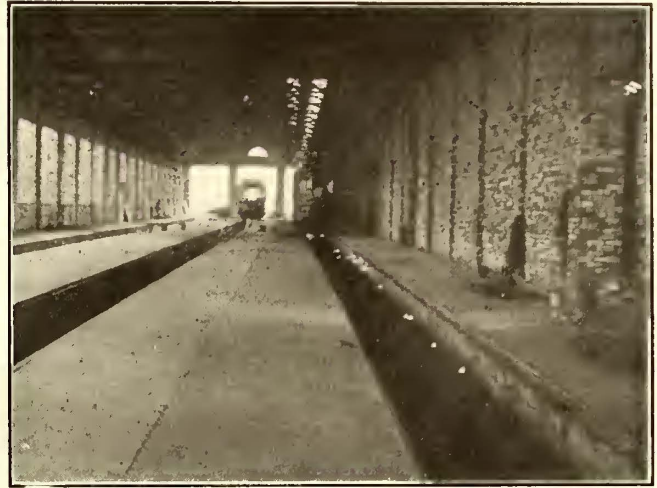
Northern Ohio Shops—East Section of Carhouse Used for Car Washing and Light Repairs
