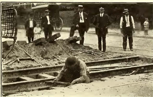
Brooklyn Joints and Ties—Sand Blasting the Rail Before Placing the Mold
