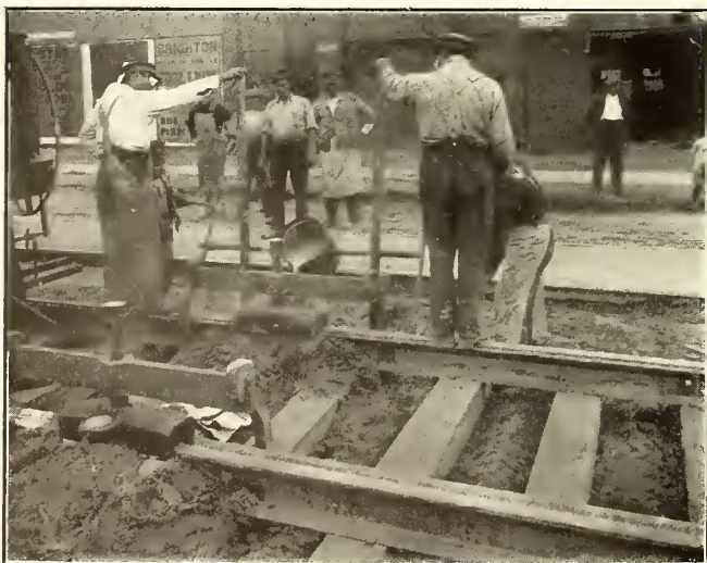
Brooklyn Joints and Ties—Pouring Cast-Weld Joint Alongside the Cupola Car
