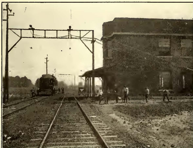
View Showing Steel Catenary Bridges and Substation on Cut-Off of Northern Ohio Traction & Light Company
