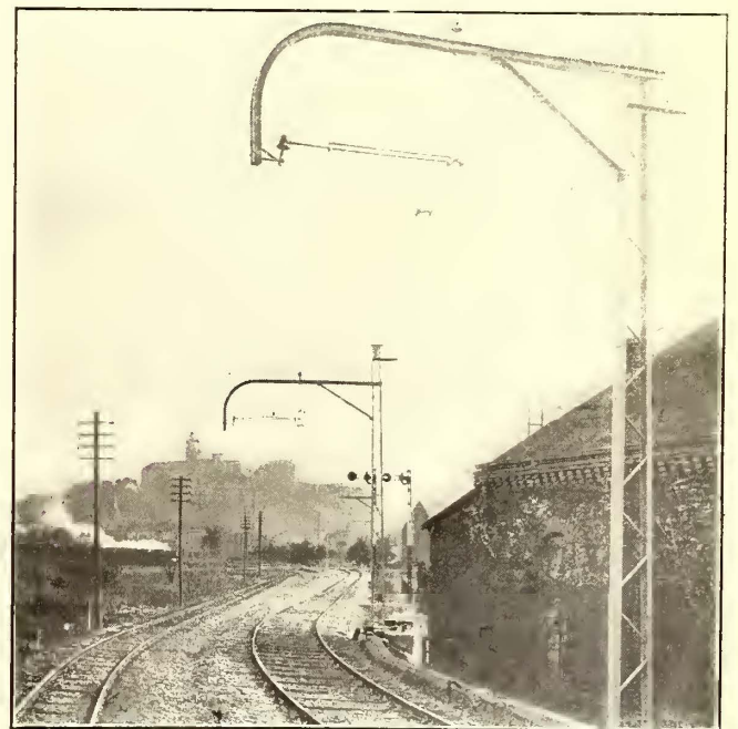
Rhine Interurban Railways—Curved Bracket Suspension on Bonn-Siegburg-Königswinter Line
