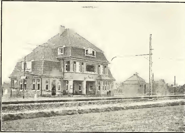
Rhine Interurban Railways—Combined Residence and Railway Station at Hangelar
