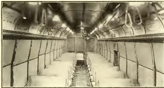
Toledo Lighting Tests—Interior View—Test B, 36-Watt Lamps with Reflectors
