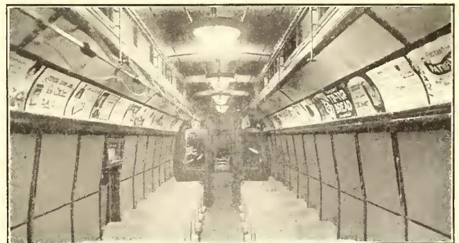
Toledo Lighting Tests—Interior View—Test F, Semi-Indirect Lighting
