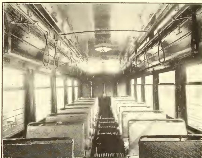
Electric Railway Car Lighting—Typical Unsatisfactory and Inefficient Lighting Arrangement
