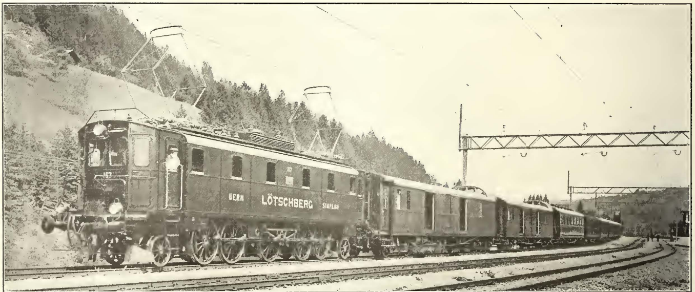
Löttschberg Locomotives—A Train in Service, Showing Also Catenary Overhead Construction
