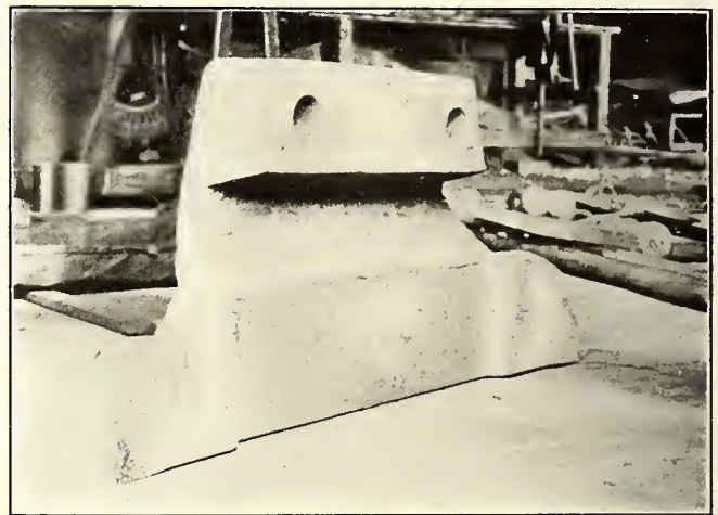
Cincinnati Track Construction—Double-Sheared Plow Casting Used to Remove Concrete Beam from Rail
