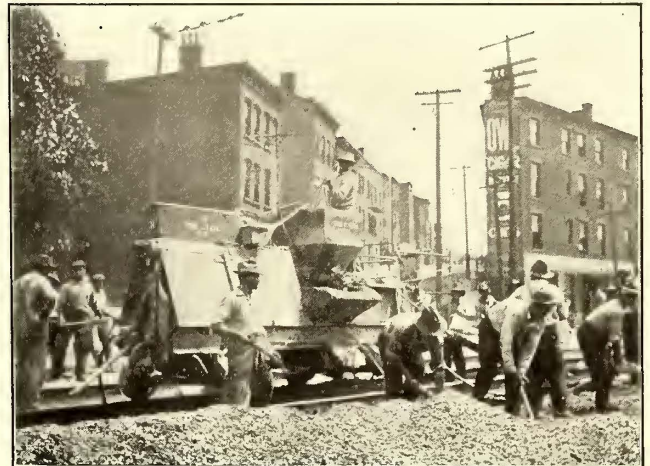
Cincinnati Track Construction—Charging End of Concrete Mixer
