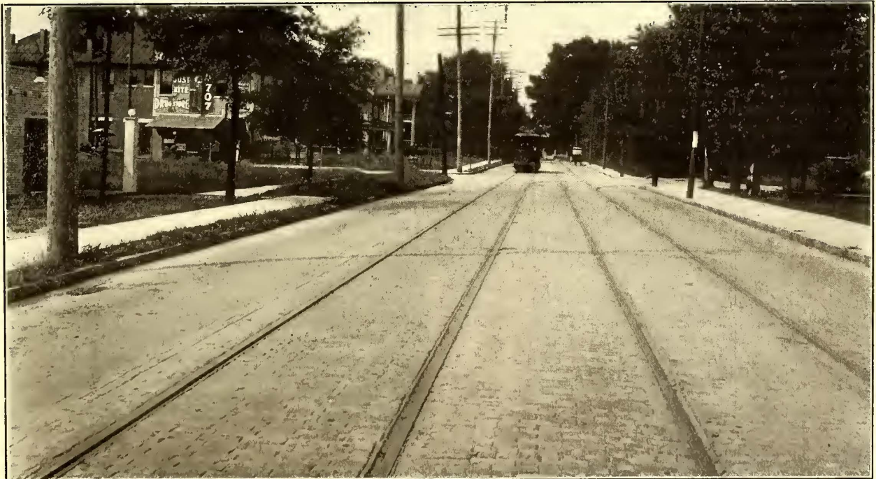
80-lb. A. S. C. E. T-Rail in Brick Paving with Paving Protector in Flangeway
