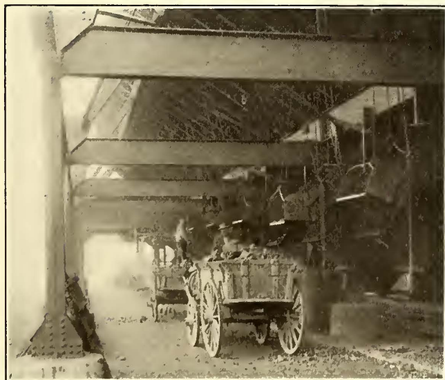
I. T. S. Coal-Handling Plant—Loading Spouts Underneath Bridge
