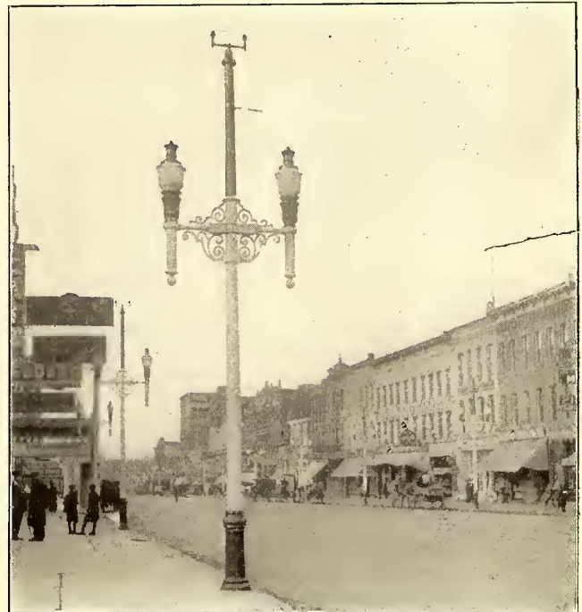
Combination Lighting and Trolley Pole
