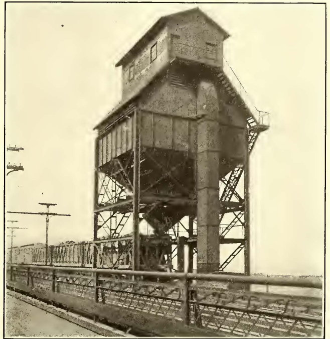
I. T. S. Coal-Handling Plant—Reloading Tipple as Seen from Bridge Deck
