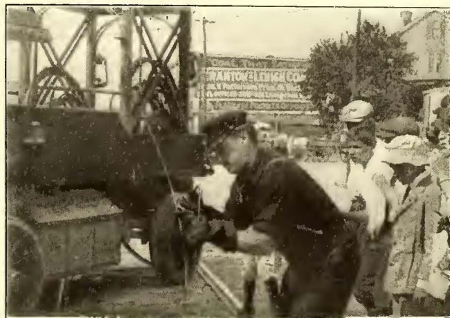
Brooklyn Accident Campaign—The Lineman Makes the Repair but Is Careful to Use Rubber Gloves
