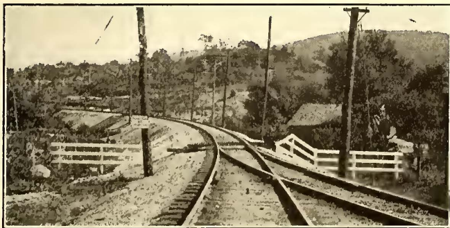
Berkshire Improvements—Beginning of Heavy Track and Roadbed Construction on Lee-Huntington Extension
