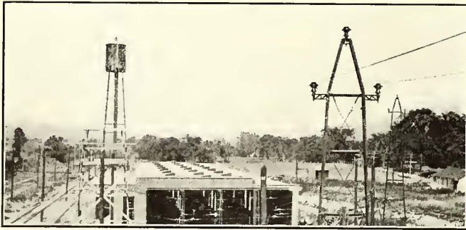
Berkshire Improvements—Sheffield Carhouse and Incoming 33,000-Volt Line
