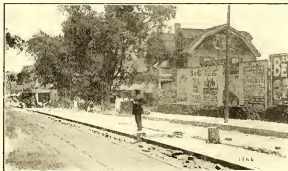
Welded Joints Left to Cool with Molds in Place.
