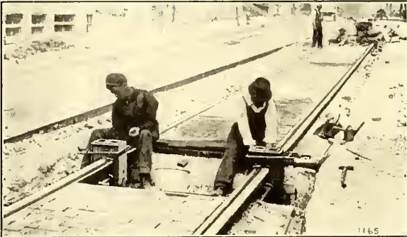
Molds as Adjusted Being Luted for Insert Rail Welds.
