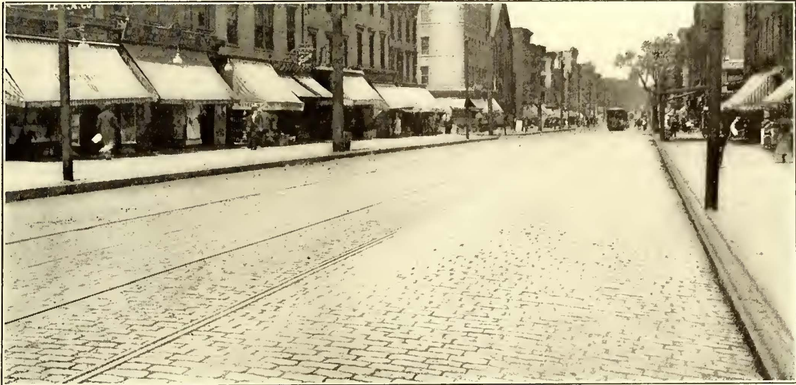
Manhattan Avenue, Brooklyn, looking east from Kent Street. Granite blocks filled with Barrett's Paving Pitch.
