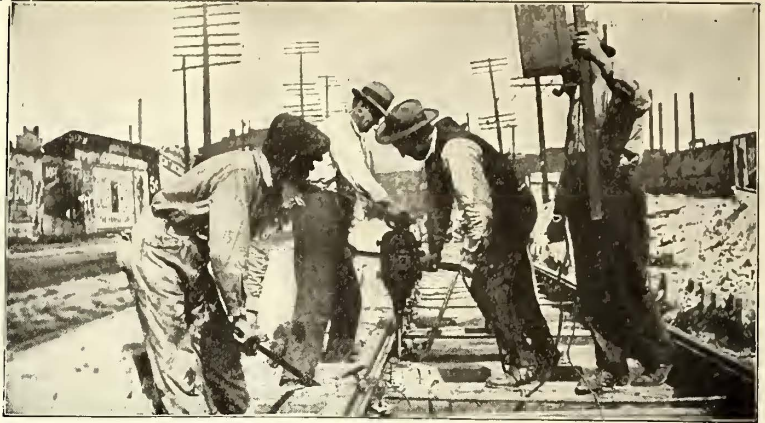
Drilling Bonding Holes with Duntley Electric Track Drill on United Railways of St. Louis
