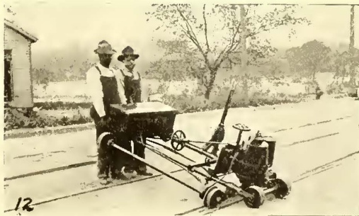
The Indianapolis Portable Electric Grinder for Resurfacing Track
