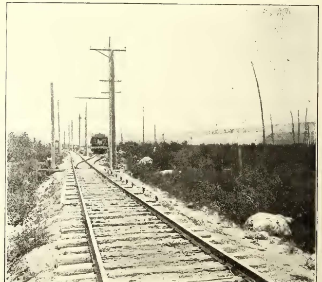
Mesaba Railway—View Showing Siding and Contact Rails for Signal System
