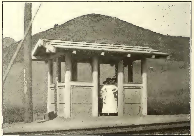
Pacific Electric Shelters—View of Completed Building, Except for Setting of Window Frames and Door
