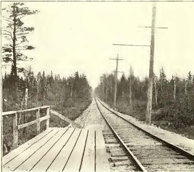
Mesaba Railway—General View Showing Character of Country and Construction
