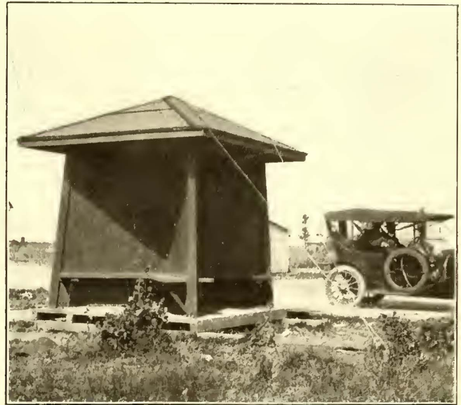
Mesaba Railway—Typical Way Shelter
