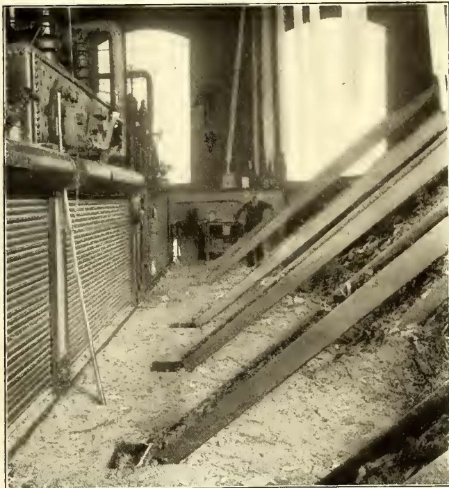
Mesaba Railway—Fuel Deck Over Boiler Room Floor
